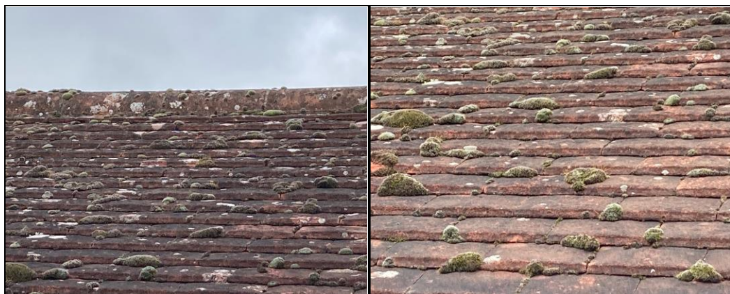
Photographs 19 - 20: Roof tiles & ridge
