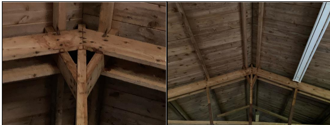
Photographs 36 - 37: Narrow rafters & wooden lining
