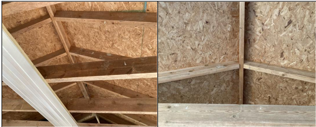
Photographs 47 - 48: Narrow rafters & wooden lining
