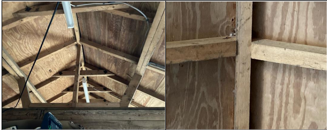
Photographs 25 - 26: Central ridge beam & wooden boarding
