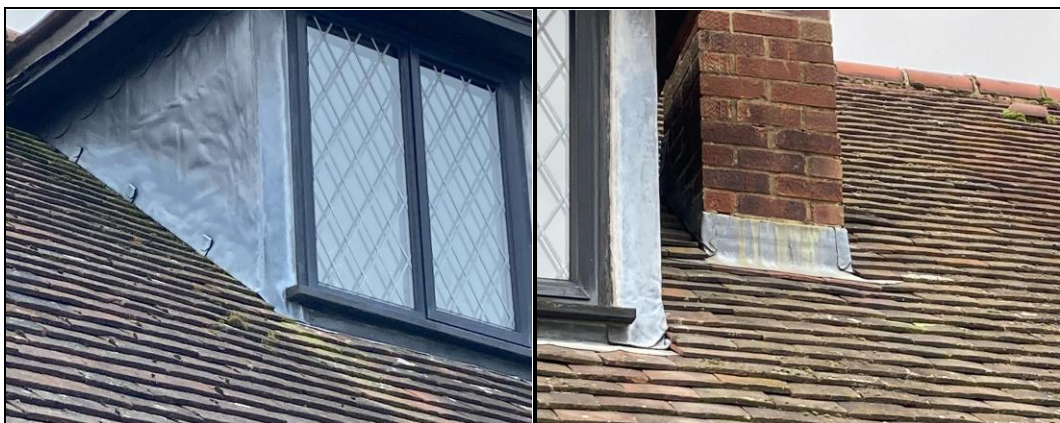
Photographs 5 - 6 : Close-fitting dormer flashings and chimney
