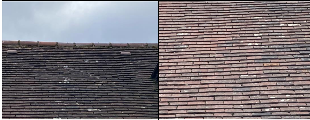
Photographs 7 - 8: Roof tiles & ridge
