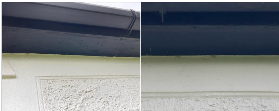
Photographs 9 - 10: Typical tight-fitting eaves/barge boards/soffits
