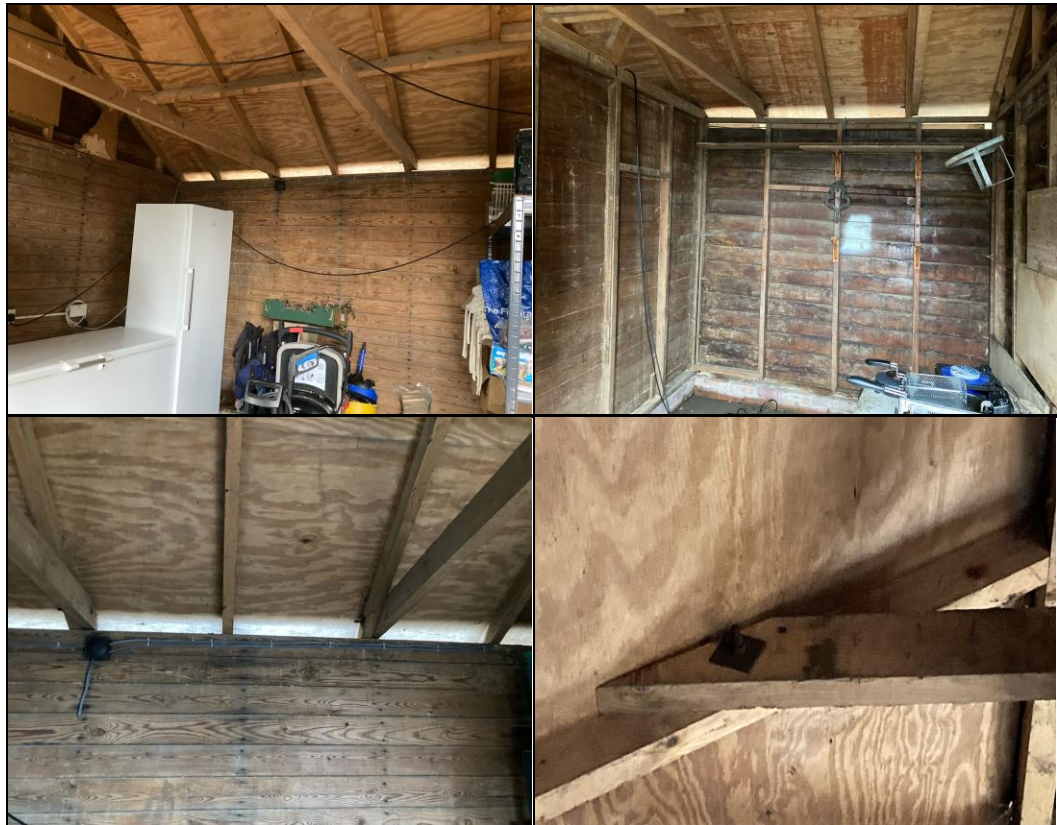
Photographs 21 - 24: Internal roof void
