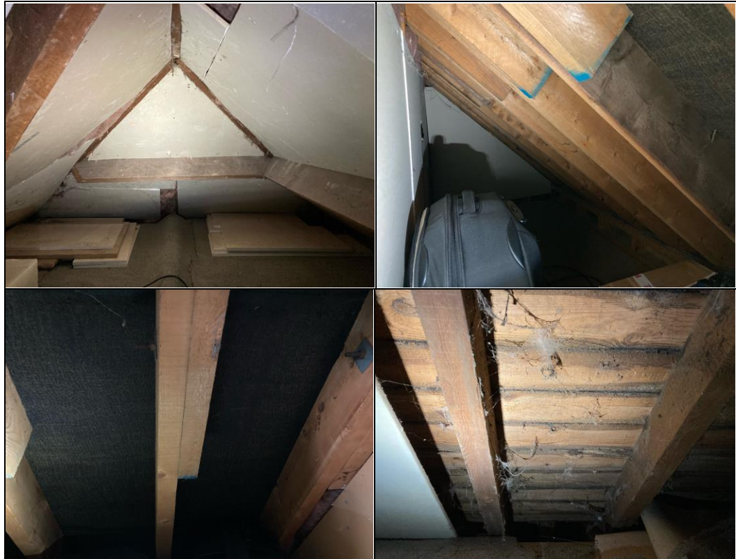
Photographs 11 - 14: Internal roof voids at eaves
