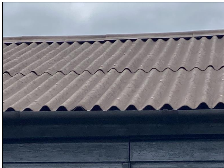
Photograph 31 : Corrugated bitumen sheet roof in excellent condition
