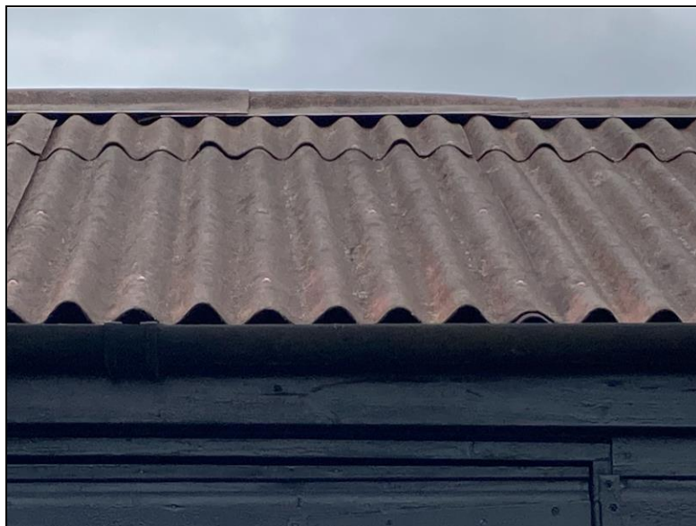
Photograph 42 : Corrugated bitumen sheet roof in excellent condition
