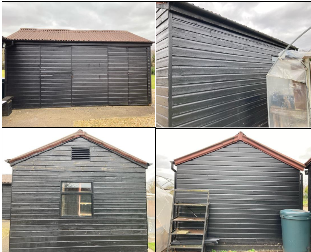
Photographs 38 - 41: Front, rear & side elevations
