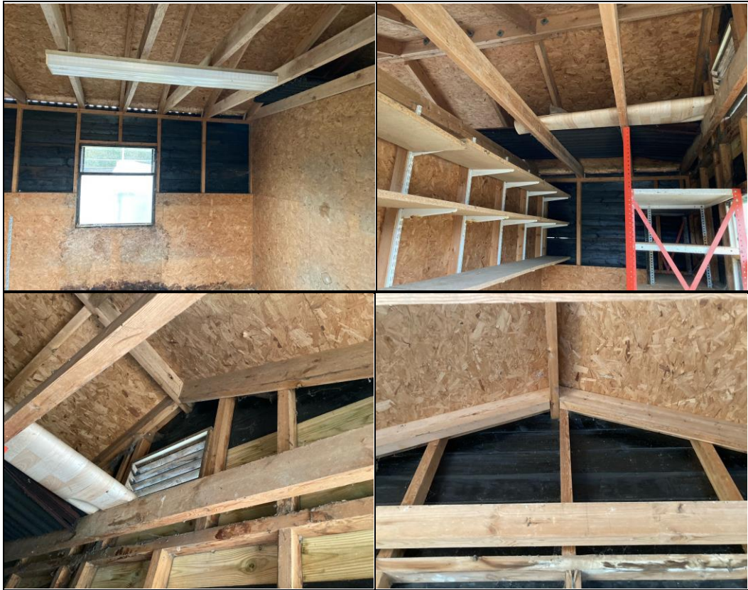
Photographs 43 - 46: Internal roof void
