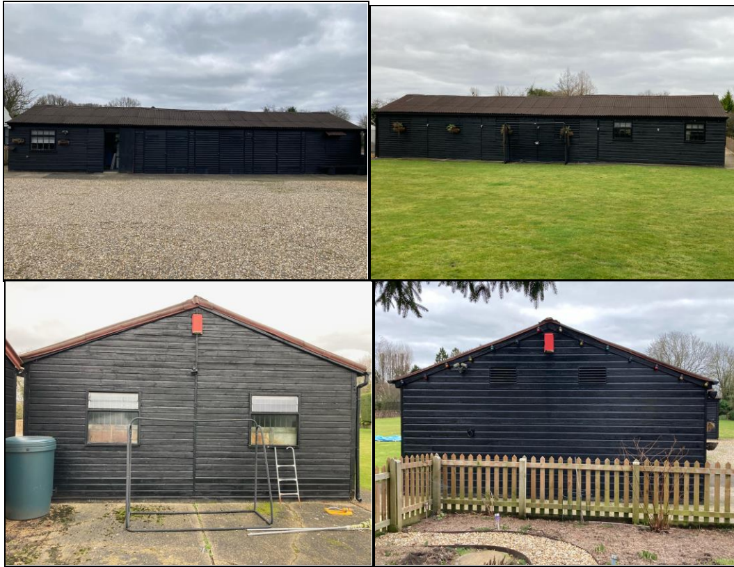
Photographs 27 - 30 : Front, rear & side elevations
