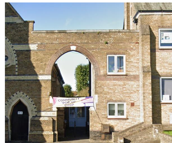
Top left: poor quality kitchen and toilet block which connected to the former schoolroom
