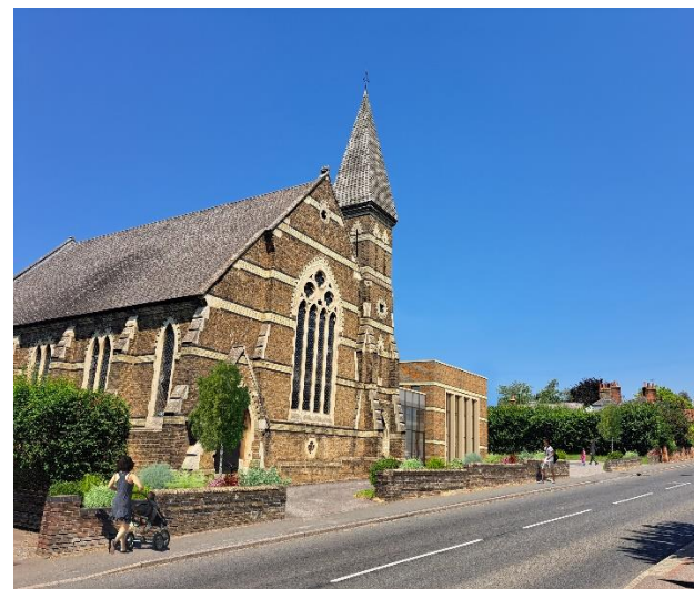
View looking northeast along London Road
