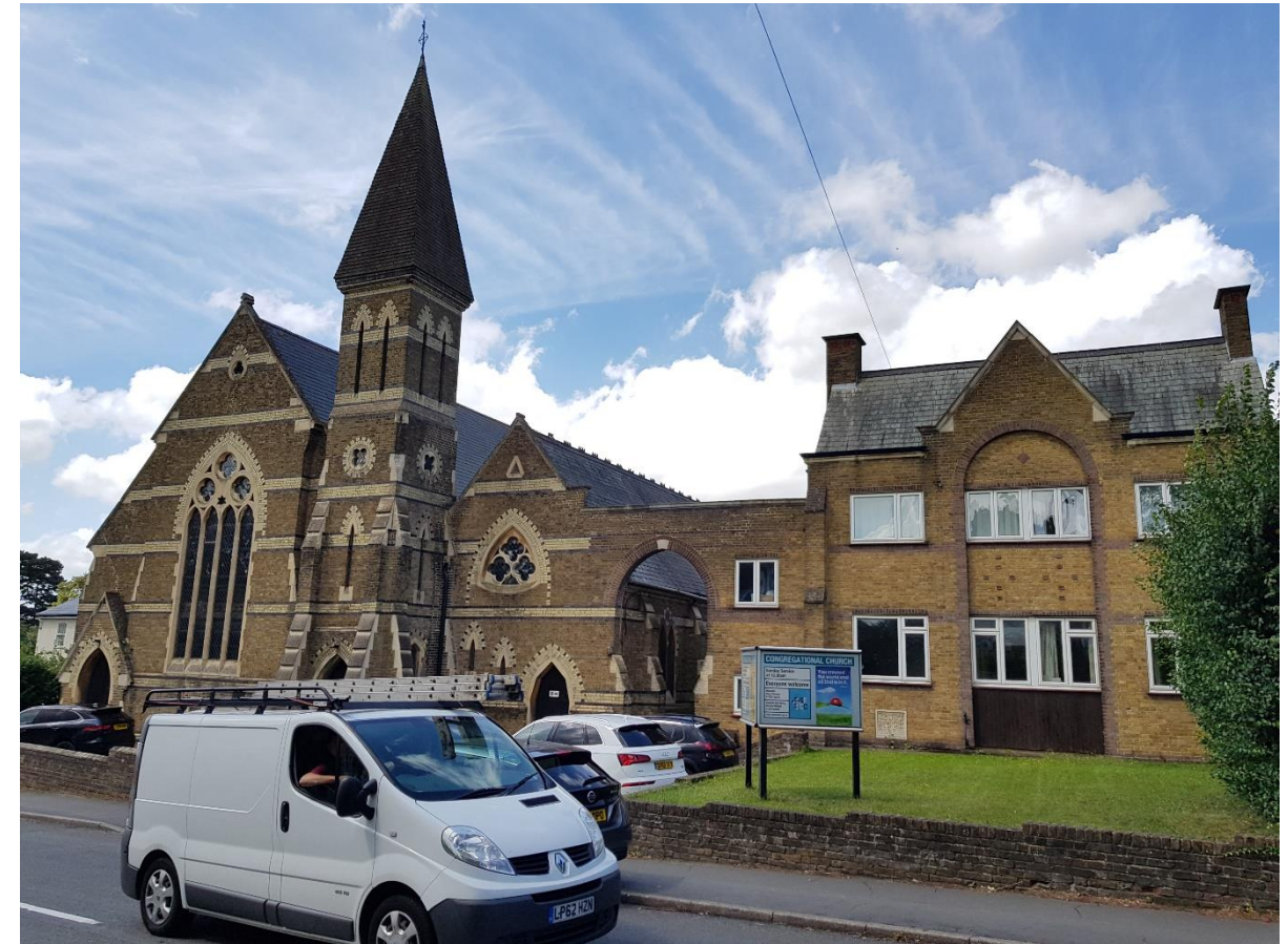
Sawbridgeworth Evangelical Congregational Church as seen from London Road (existing view)
