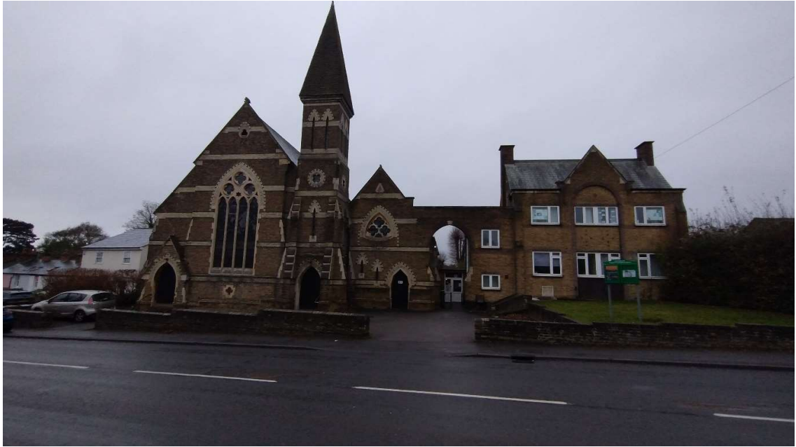
Figure 2 Frontage of SEC Church on London Road.
