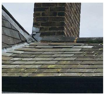
Repairs needed: clean down and remove moss from roof and rebed ridge tile with new mortar.
