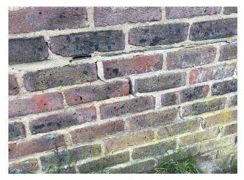
Repairs needed: repoint areas of missing mortar around DPC.
