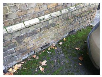
Repairs needed: carry out patch pointing to the lower levels to the brick plinths at low level to the wall as required.
