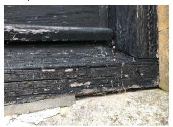
Repairs needed: repoint around timber frame and replace rotten sub-cill and redecorate window entirely.
