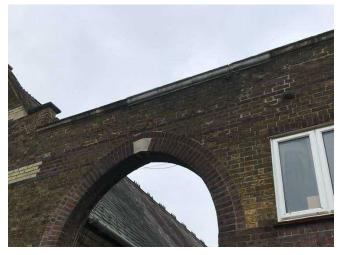
Repairs needed: clean back plant growth and repoint as required to brickwork and stone cappings.
