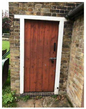
Repairs needed: redecorate doors and allow for minor repairs to the timber frame of the boiler house door at low level.
