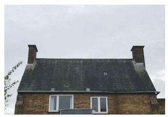
Repairs needed: replace missing tiles, rebed ridge tiles and refix any loose and slipping tiles, refix and redress lead flashings as required.
