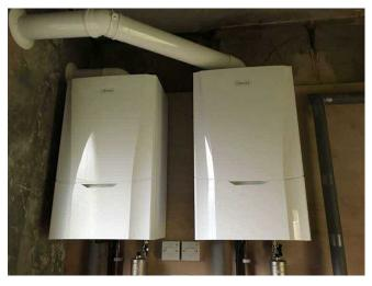
Heating system for schoolhouse: this is a conventional wet system, with the gas boiler located in the toilet cubicle on the ground floor, distributing heat around the building to steel panel radiators.
