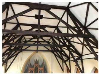
7.2 **North aisle roof structure:** a series of five high pitched timber roof trusses largely exposed. There is a high level flat section of ceiling to the apex. All ceiling panels between timbers appear to be a plastered finish, presumably of lath and plaster. Close access to the roof structure is not possible.
