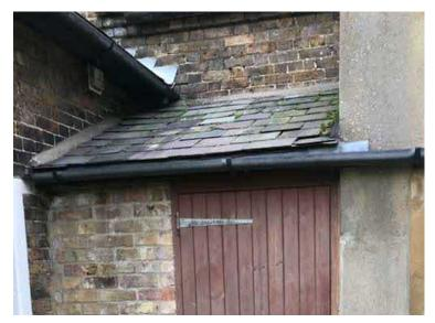
Repairs needed: replace deteriorated slates.
