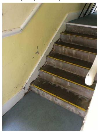
Repairs needed: clean back walls where surface deterioration has occurred and redecorate using a breathable paint.
