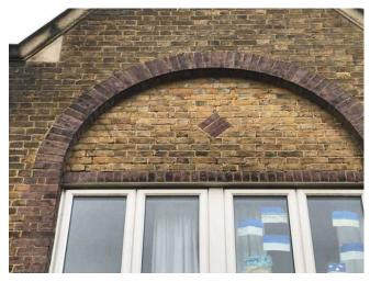
Repairs needed: replace deteriorated stone and allow to repoint areas of missing mortar across the brick elevations.
