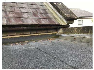
2.6 **External storage room next to vestry tollet:** a natural slate roof laid with a random mix of different types of slates, several of which appear to be old re-used slates, with mortar fillets at abutments to walls.
