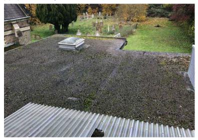
Repairs needed: replace felt covering to flat roof and allow to replace areas of rotten decking board beneath and allow for minor structural repairs, depending on findings once works begin.
