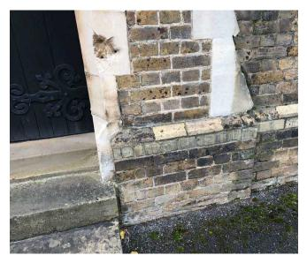
Repairs needed: carry out repointing at low level to the brickwork and pare back soft areas of stone and apply a lime shelter coat.
