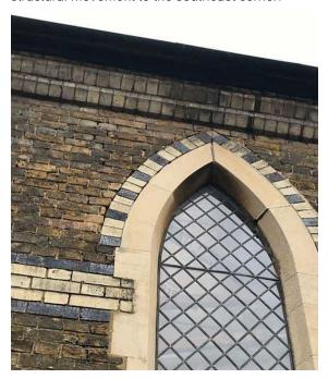
Repairs needed: carry out repointing to east over stone window arch and monitor minor cracking for further movement.
