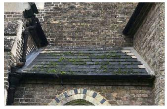
Repairs needed: clean down roof covering and remove moss to prevent blocking-up of gutter.
