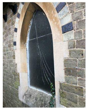
Repairs needed: replace glass.
