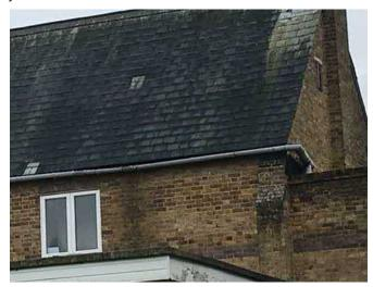
Repairs needed: clean, reseal joints and redecorate cast iron gutters and refix uPVC guttering to the rear to provide adequate falls.
