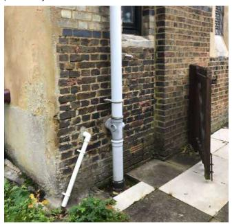
Repairs needed: repoint brickwork to south wall and re-render wall to west.
