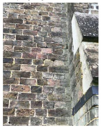
Repairs needed: carry out patch pointing where required.
