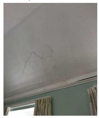
Repairs needed: remove sections of ceiling and inspect the timber roof structure behind and gain access to the higher roof void for further closer inspection of the roof timbers and allow for a level of repair to the roof timbers and replacement if required.
