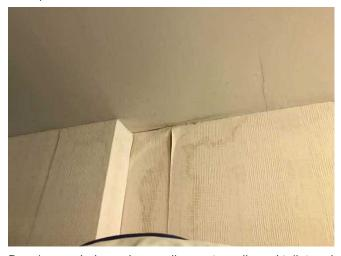
Repairs needed: replace wallpaper to walls and toilet and allow to replaster where leaks have damaged prior to redecorating or reapplying wallpaper.
