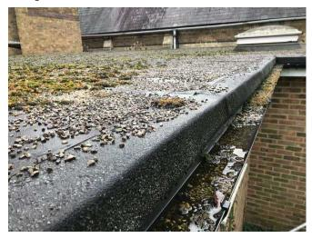
Repairs needed: clean out gutters and downpipes.
