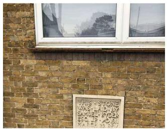
4.20 Repairs needed: repoint cracks and monitor for further movement, with the clay tile cill being repaired.
