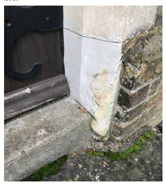
Repairs needed: remove poor quality historic repair to stone reveal and apply lime shelter coat throughout.
