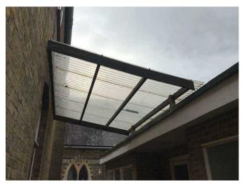
Repair needed: clean down canopy and replace damaged section.
