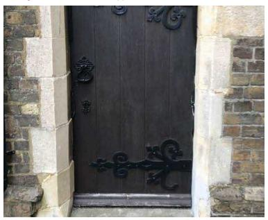
Repairs needed: redecorate door and ironmongery and replace sealant around door.
