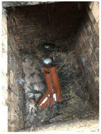
Repairs needed: clean through the foul drainage system and have a CCTV survey carried out to ensure it is in good condition and remove any roots within the manhole or drainage system.
