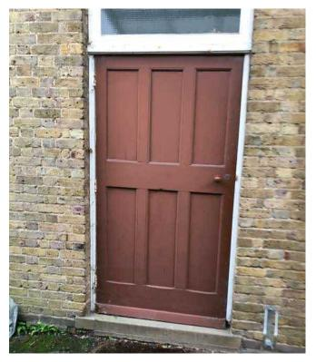
Repairs needed: redecorate door and apply timber repair to weather strip.
