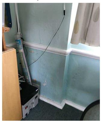
Repairs needed: as included in roof structure section, damp sections to the walls should have the plaster removed and replaced and redecoration carried out once the source of water externally has been removed and repaired.
