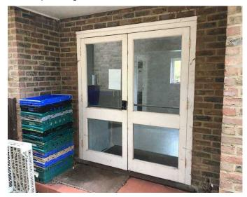
Repairs needed: redecorate, including ironmongery, and replace cracked pane to door.
