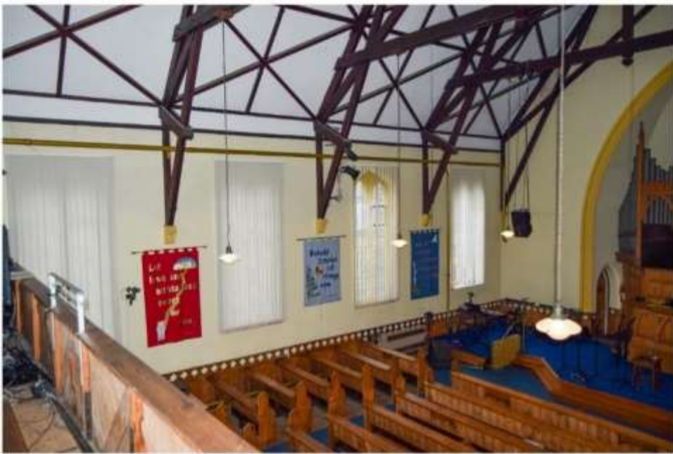
iii) Looking southwest
