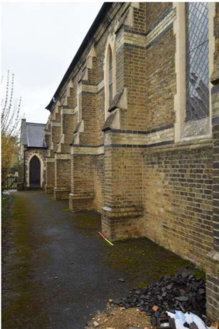
v) buttress details on south elevation
