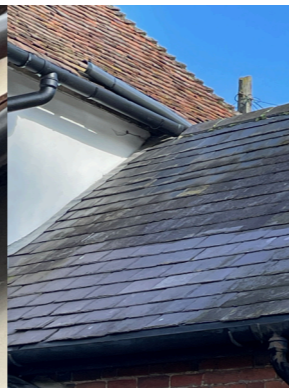
Roof abutment viewed from west
