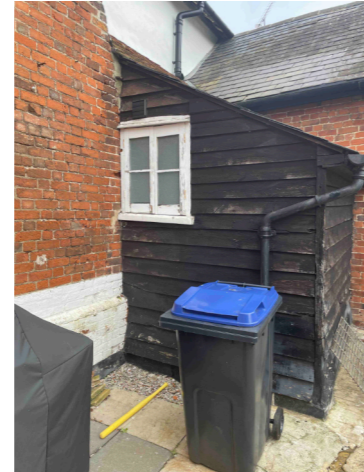
Existing ground floor bathroom
