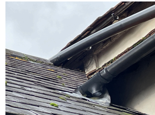
Roof abutment viewed from east
