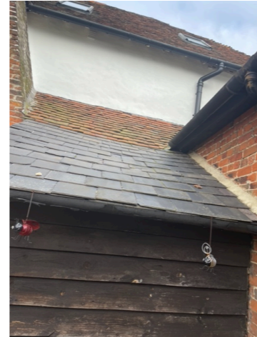
Existing roof over bathroom
