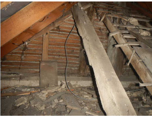
Junction of rear range roof with roof of The Angel
