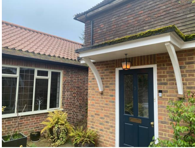
Flat roof porch added under PLAN/2014/0127
