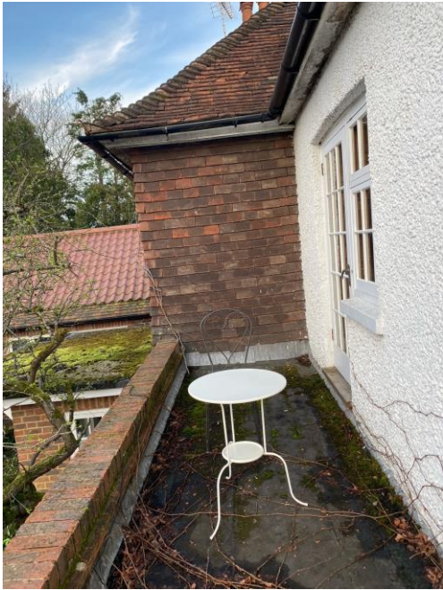
Balcony looking NE
