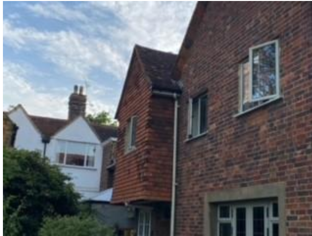
Rear elevation – example of the variety of materials
