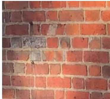
Red brick with lime mortar
