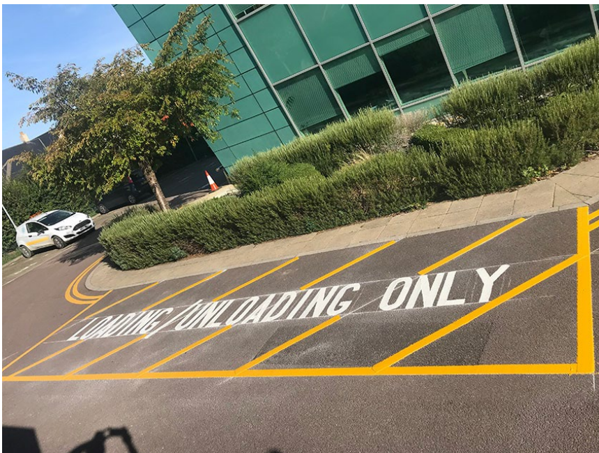
Figure 4 Loading Bay Marking (Source: www.roadartltd.co.uk )
