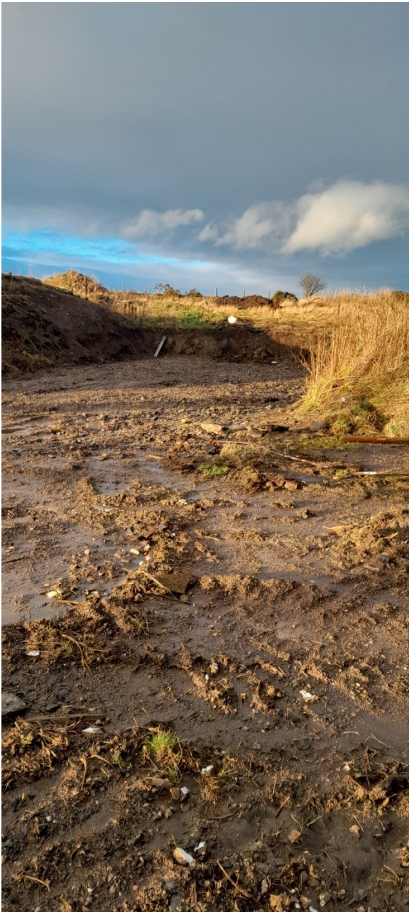
Fig 1 Cleared Site Looking North
