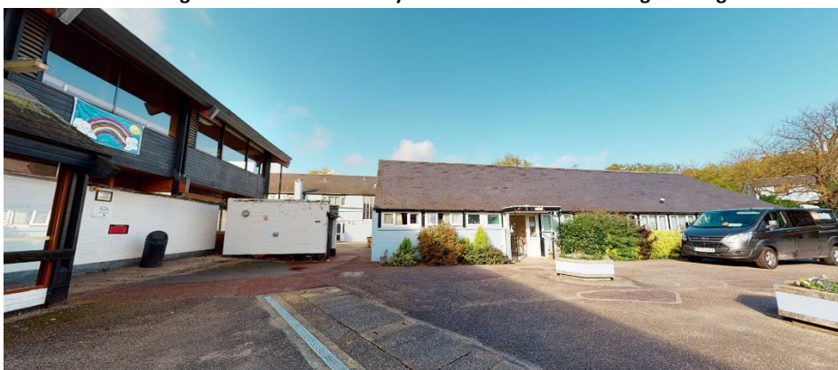
Image 3 – internal site courtyard view of the surrounding building
