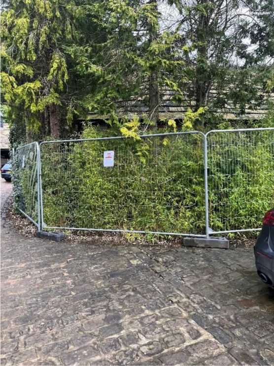
Photo 5. Further photos of Tree Protection Fencing along G2.
