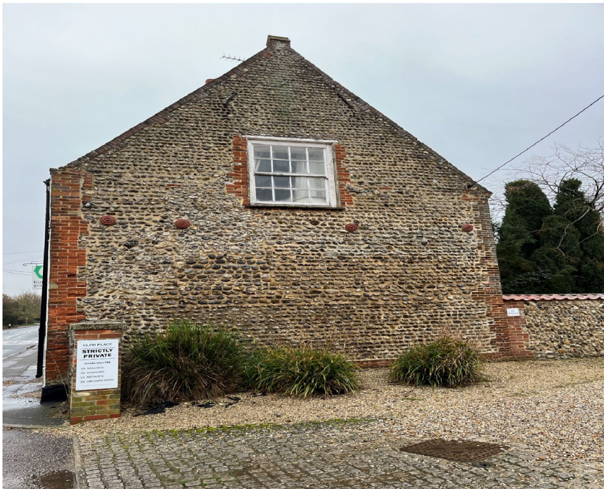
WEST GABLE NOT AFFECTED BY THE WORKS
