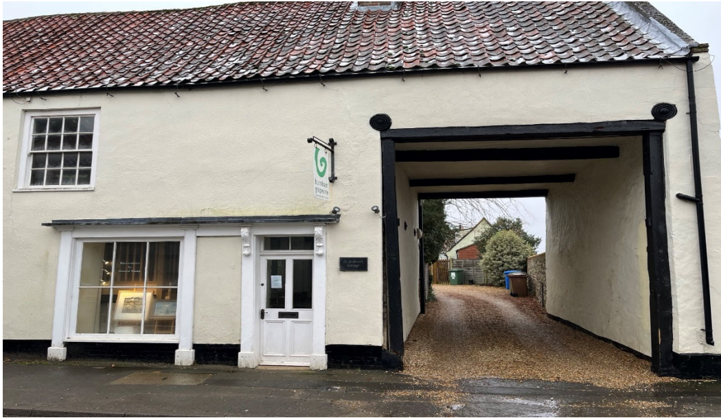
NORTH ELEVATION NOT AFFECTED BY WORKS – ENTRANCE TO REAR CAR PARK
