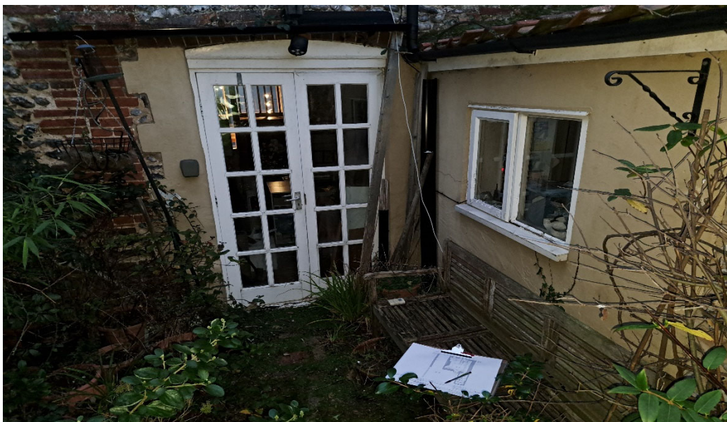
EXISTING SINGLE STORY EXTENSION BEING DEMOLISHED
