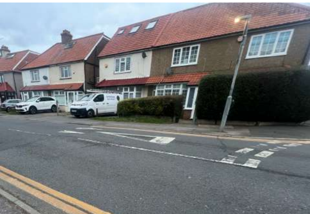
Photo 3: Existing drop kerb at 370 Gander Green Ln
