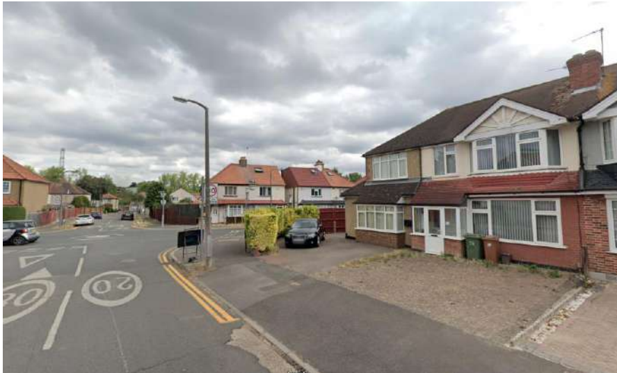
1 Brocks Drive, Parking at the front of the property accessed from kerb in close proximity to road junction between Brocks Drive and Gander Green Lane
