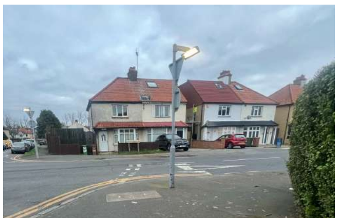
Photo 4: Existing drop kerb at 368 Gander Green Ln
