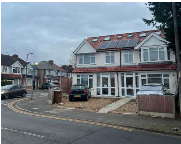
Photo 1: Existing drop kerb at 469 Gander Green Ln
