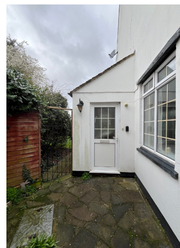
Front, side and rear of property
