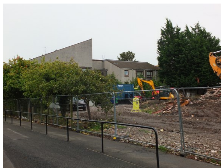
2 Rear of site with Trust Housing Association beyond
