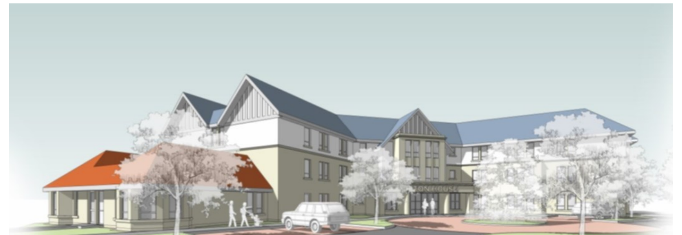
1. New care home currently under construction in Haddington.
