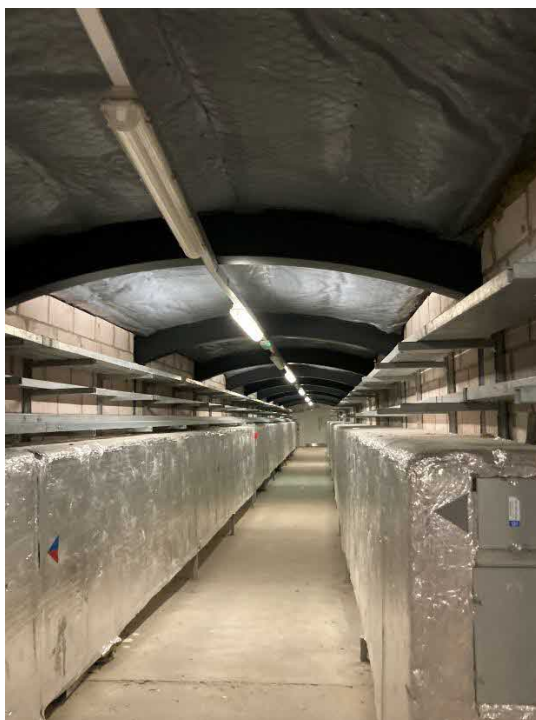
Figure 4 - Roof's build-up, photo by CK21.
