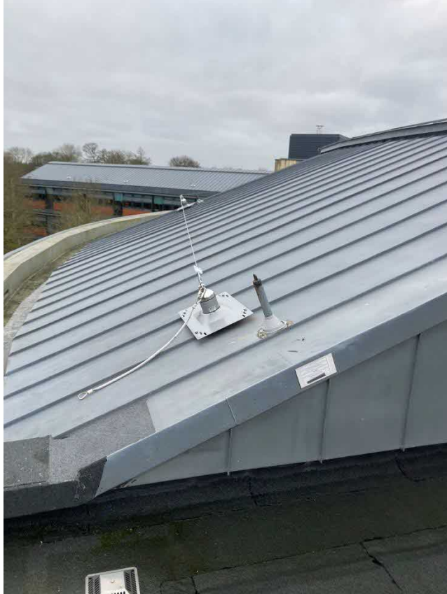
Figure 2 - Hipped roof, photo by CK21.
