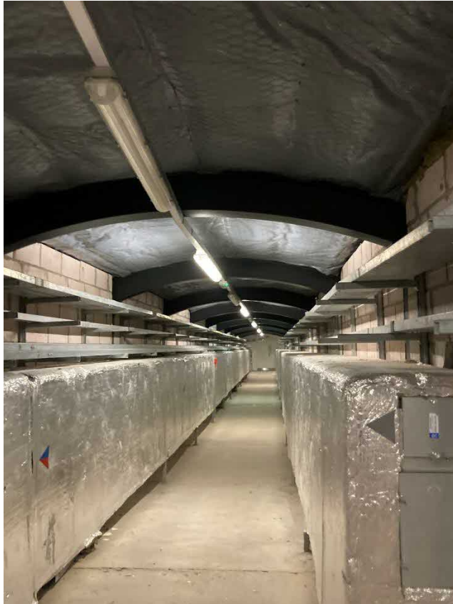
Figure 10 : Service corridor, photo by CK21.
