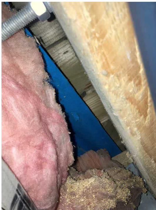
Figure 6 - Timber rafters, photo by CK21.
