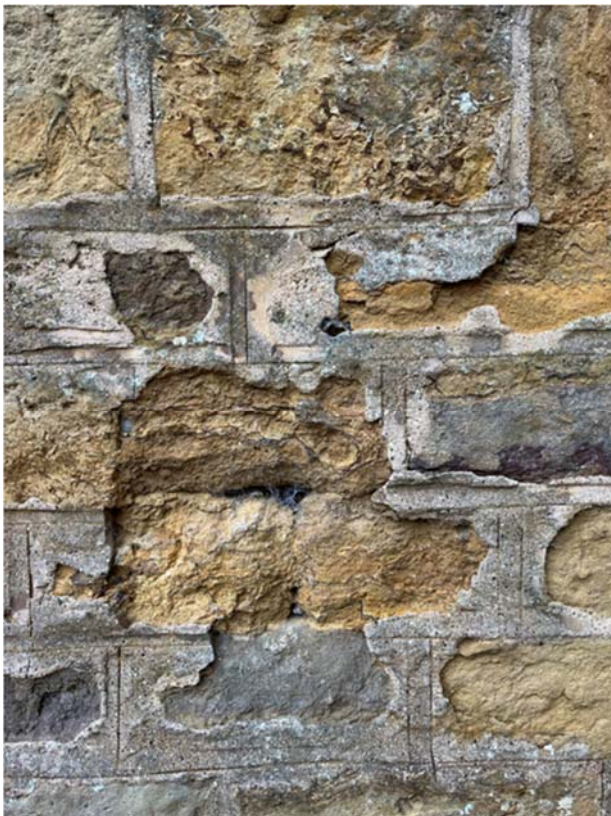
Photo 16 – Part 4 of the Work showing the condition of the gable.
