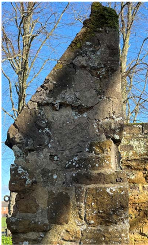
Photo 12 – Part 3 of Work Top of Wall & Capping Arrangement
