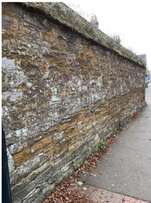
Photo 14 – Part 3 of Work – Condition of the Wall
