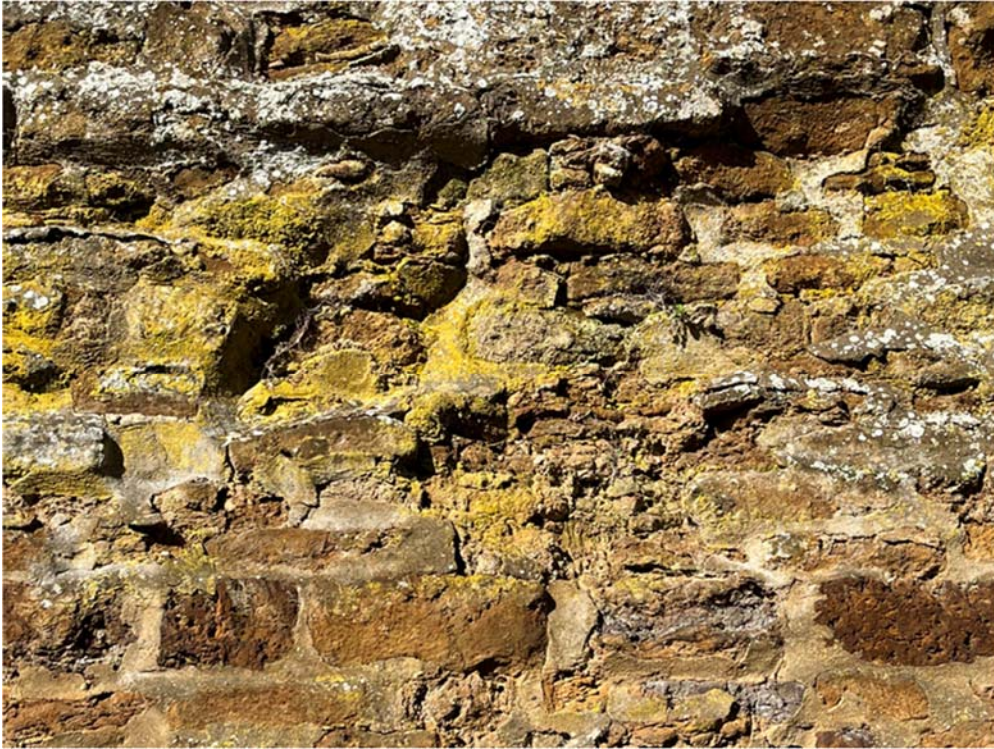
Photo 10 – Part 2 of Work - Condition of the Wall
