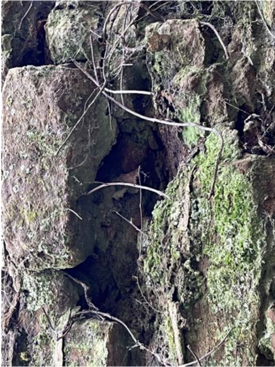
Photo 4 – Part 1 of Work – Condition of the Wall
