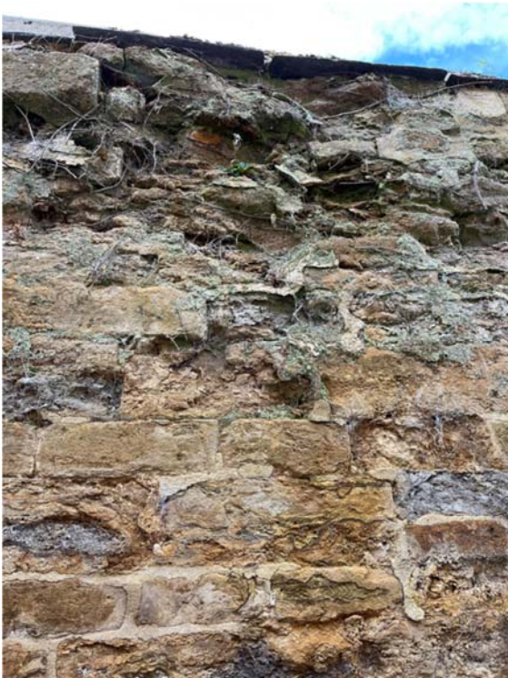
Photo 3 – Part 1 of Work - Condition of the Wall
