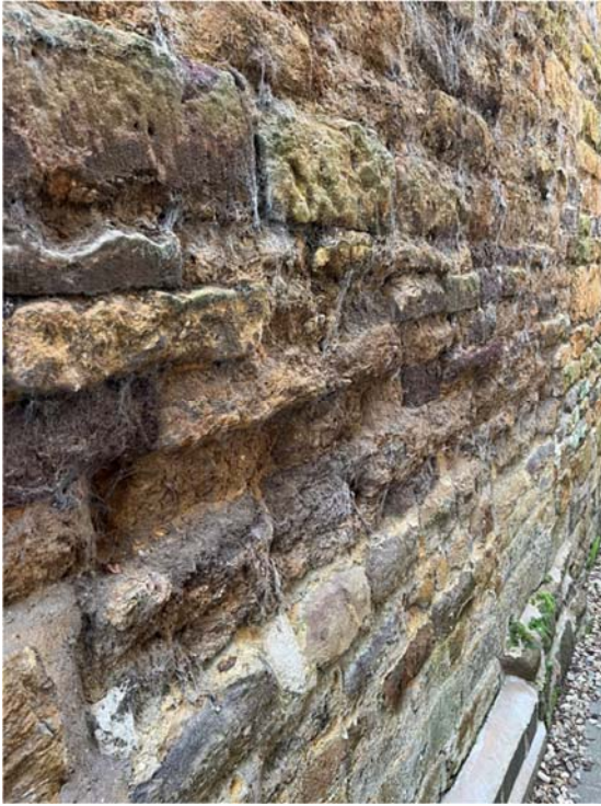
Photo 2 – Part 1 of Work - Condition of the Wall
