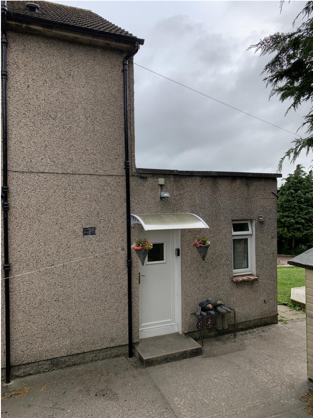
Rear of Garage/Utility (East Elevation)
