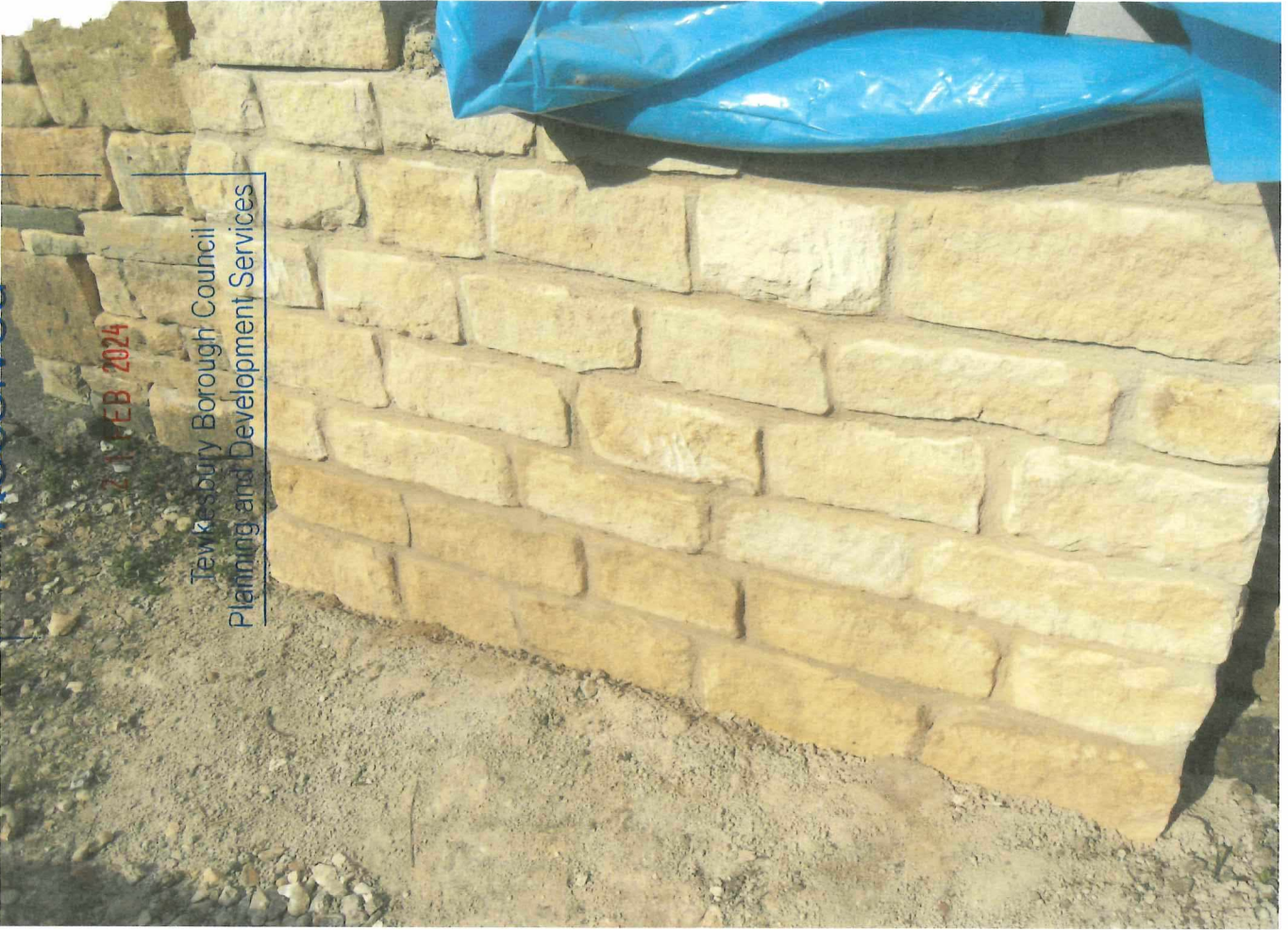
natural stone c/lime pointed (Cotswold stone) SITE PANEL
