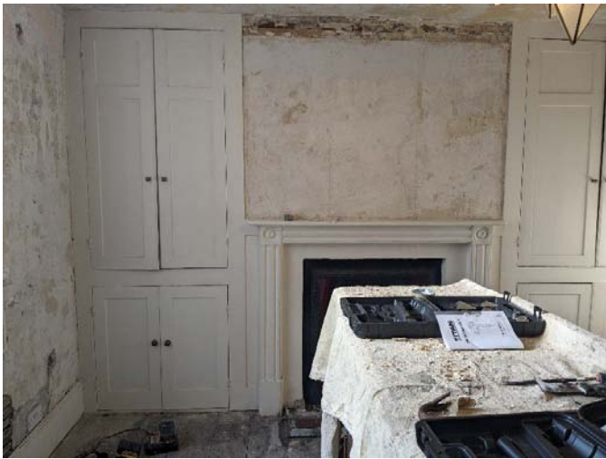
Figure 4 Existing basement front room. Note extant cupboards and floor boards.
