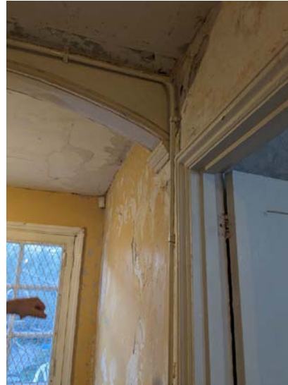
Figure 3 Existing basement area showing joinery and lathe and plaster
