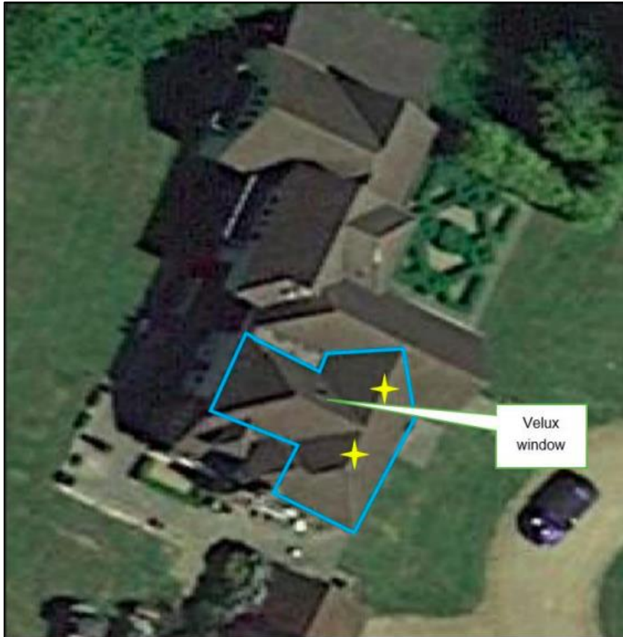
Figure 3. The roof void that was accessed is outlined in blue, confirmed brown long-eared bat roosts are signified with a star.
