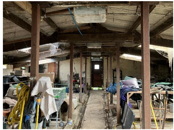
Photo 14: Internal view of Building 2
