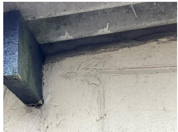
Photo 12: Closely fitting end beams and roofing sheets of B1
