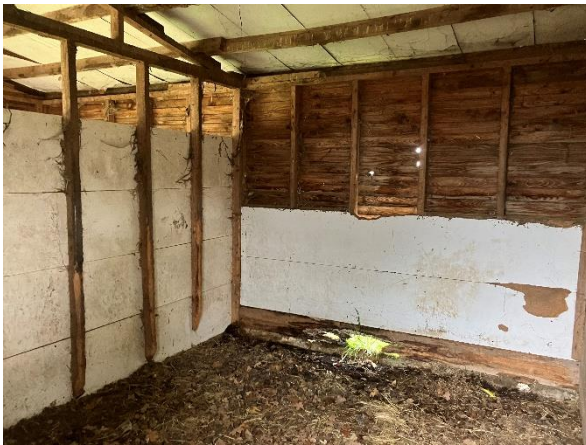
Photo 27: Internal view of Building 5
