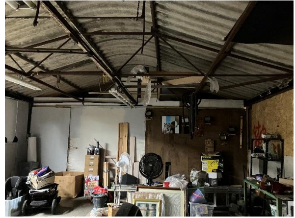
Photo 22: Internal structure of Building 4
