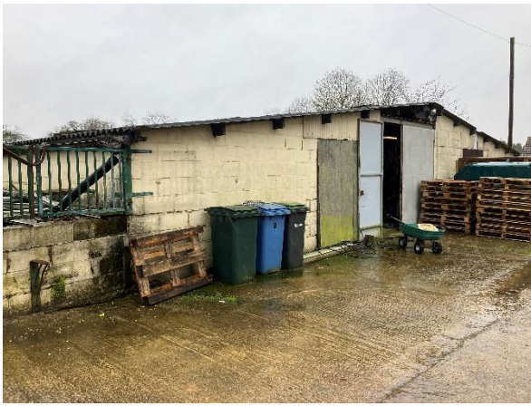
Photo 9: Northern façade of Building 1
