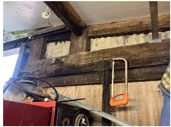
Photo 10: Internal structure of B1 – a mix of closely fitting wooden and metal supports
