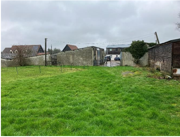
Photo 17: Southern façade of Building 3 – in centre with long sloping roof
