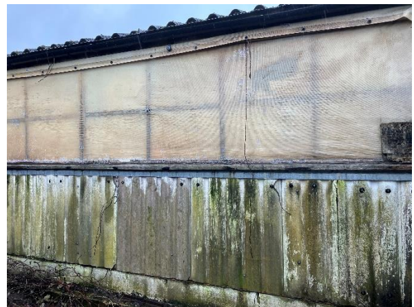
Photo 24: Eastern wall of Building 4
