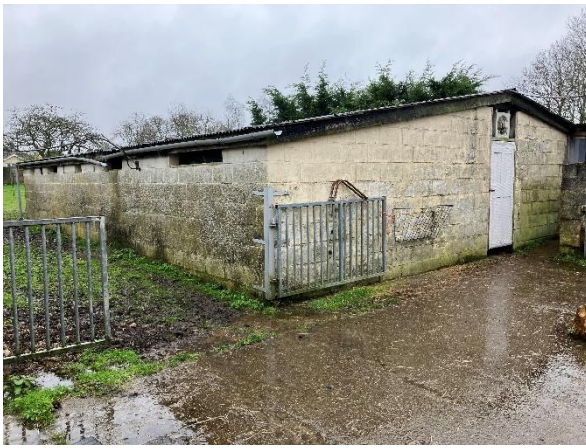
Photo 13: North eastern facades of Building 2
