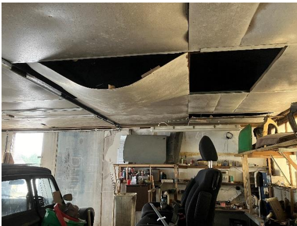
Photo 23: Metal sheet ceiling at northern end of Building 4
