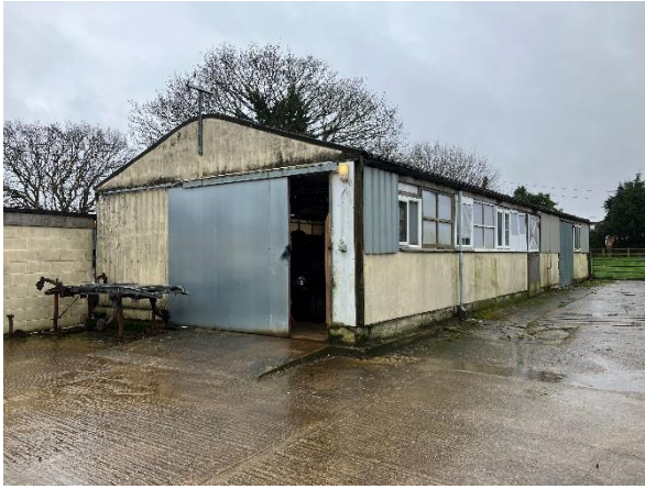
Photo 21: North western façades of Building 4
