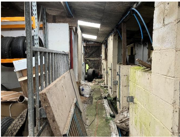
Photo 19: Internal view of Building 3
