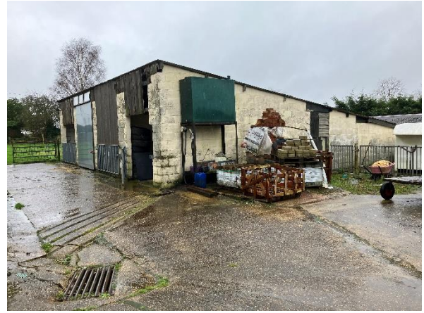
Photo 18: North eastern facades of Building 3
