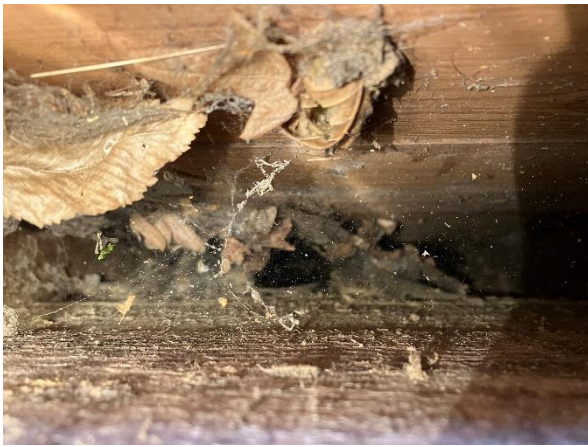
Photo 31: Typical view inside lower wall cavities
