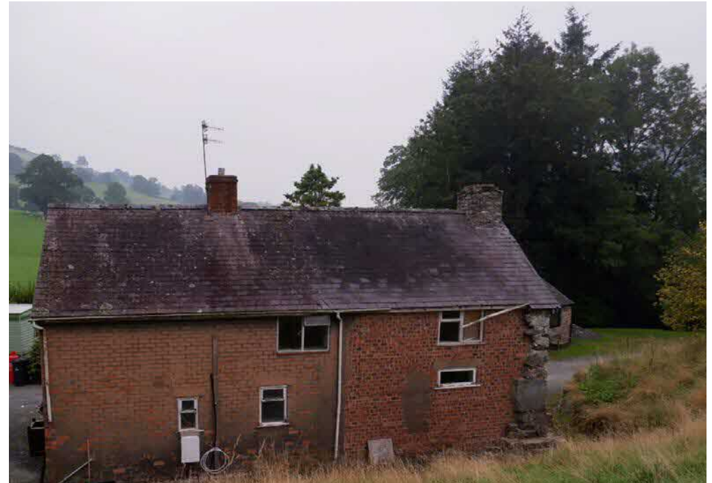
Photo of the existing house looking south-east to the main aspect from the site.
