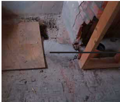
Concrete ground floor slab with no insulation
