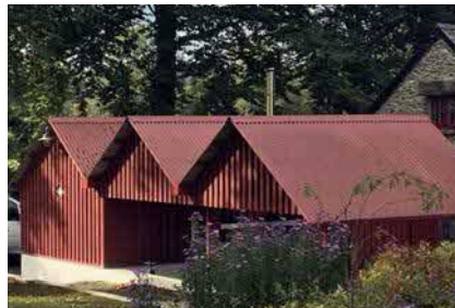
Outbuildings to stone house Rural office architects, Mid-wales
