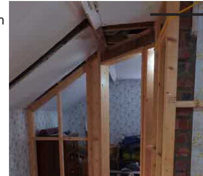
modern softwood studwork and roof. Gypsum plasterboard
