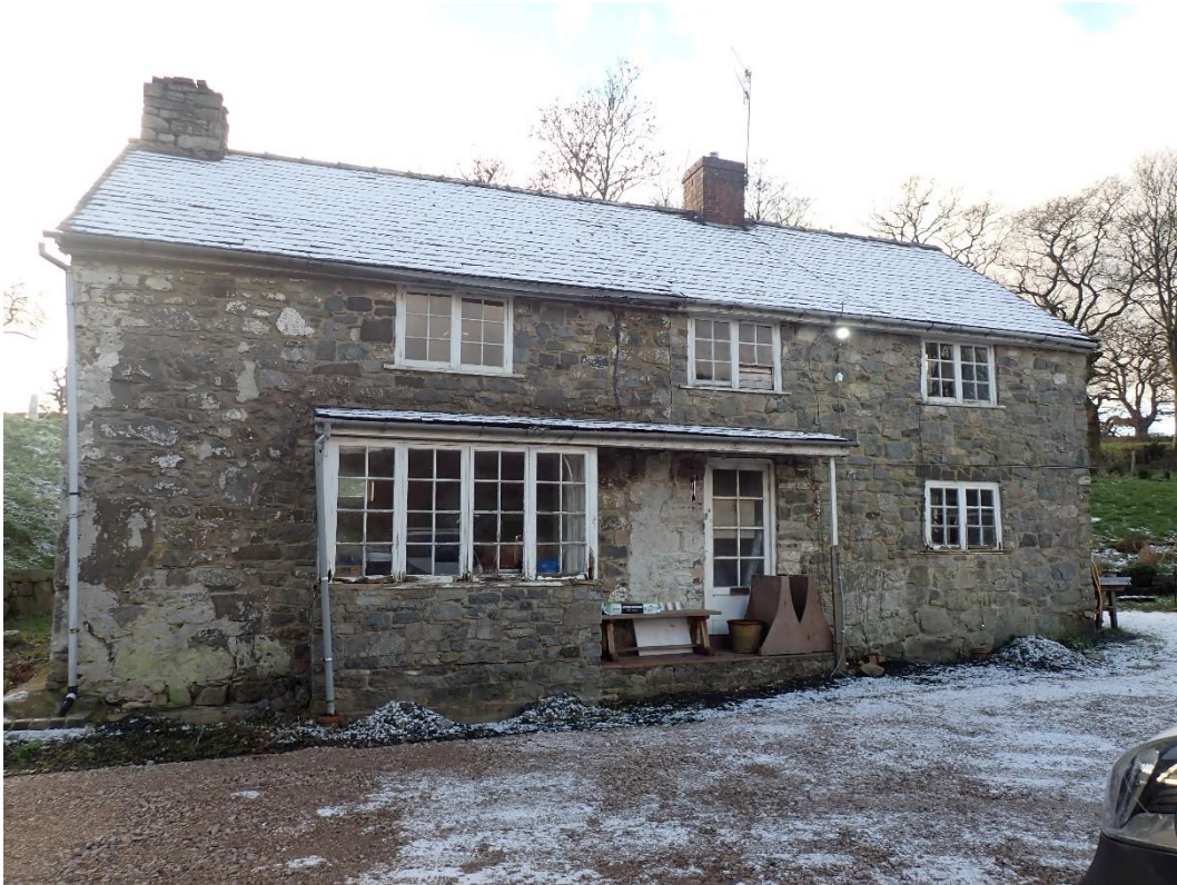
Photo 7. View of the existing dwelling which is scheduled for demolition.
