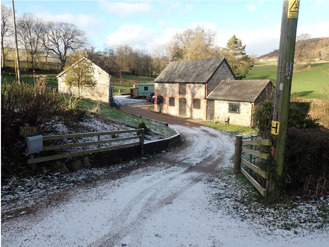
Photo 5. View from the site entrance of the existing arrangement of buildings and garden.
