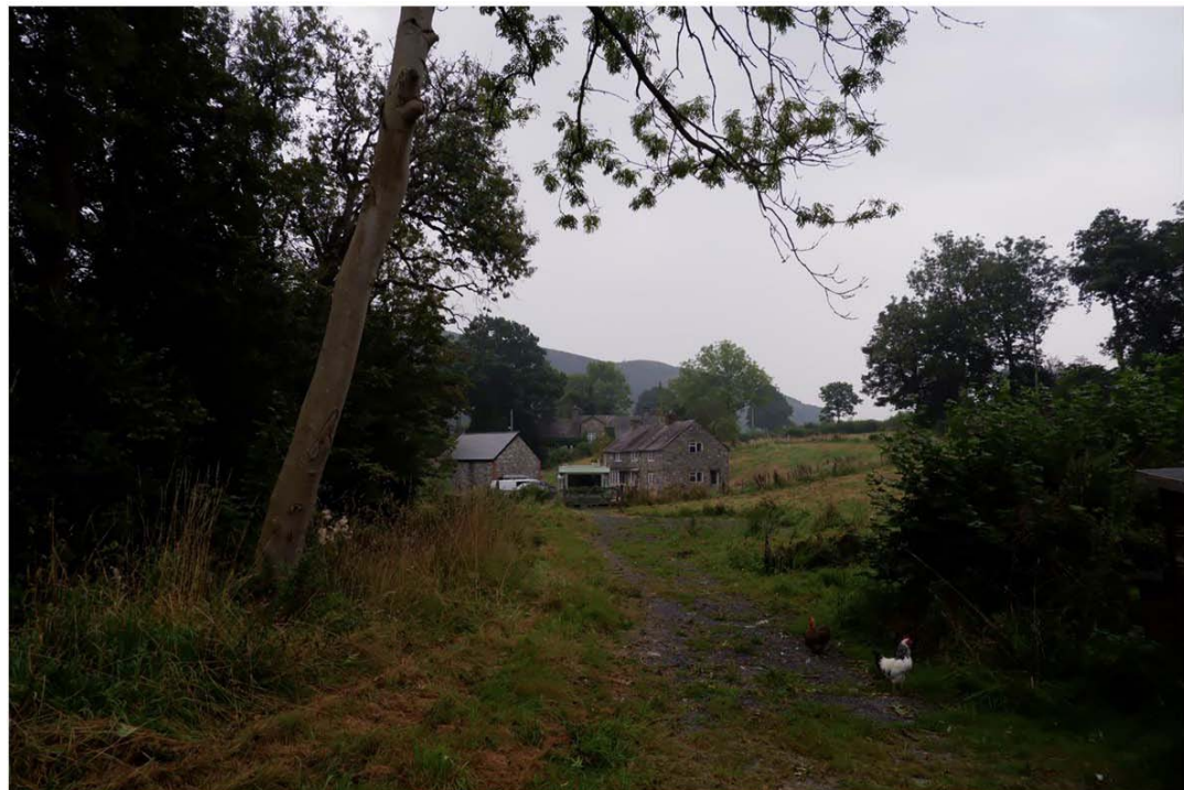
01 - Existing house and outbuilding as viewed from north
