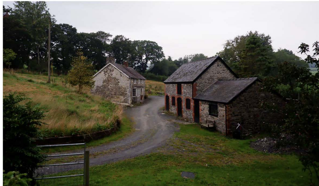
02 - Existing house and outbuilding as viewed from south
