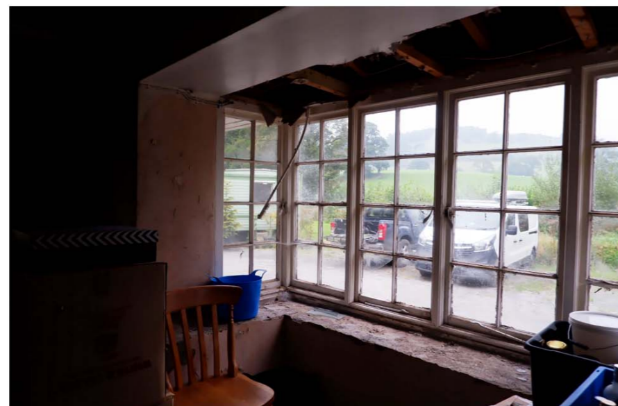
22 - Bay window - living room
