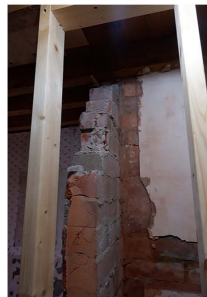
23 - Bathroom internal wall
