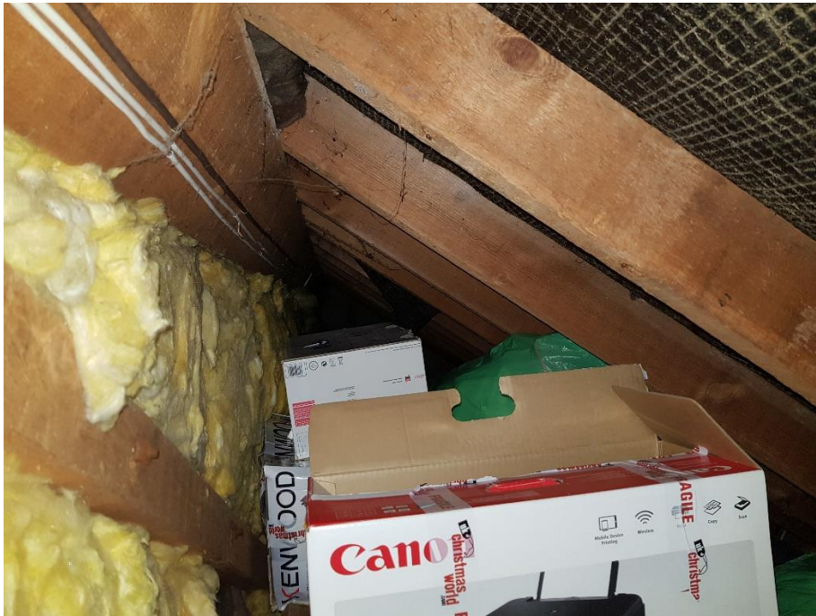
Plate 3 - Internal loft space of the house (B1)
