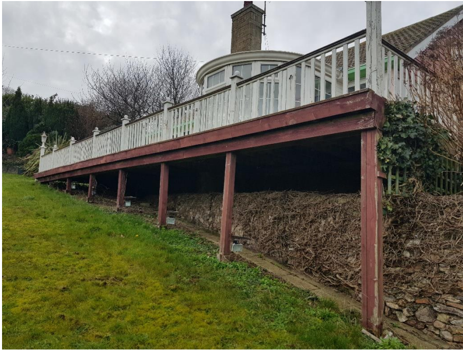
Plate 11 - West-facing view of the decking and the area underneath the decking
