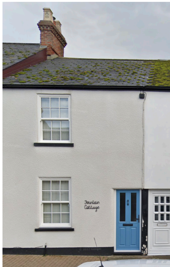
Clipped eaves is a traditional detail that can be seen in Beer
