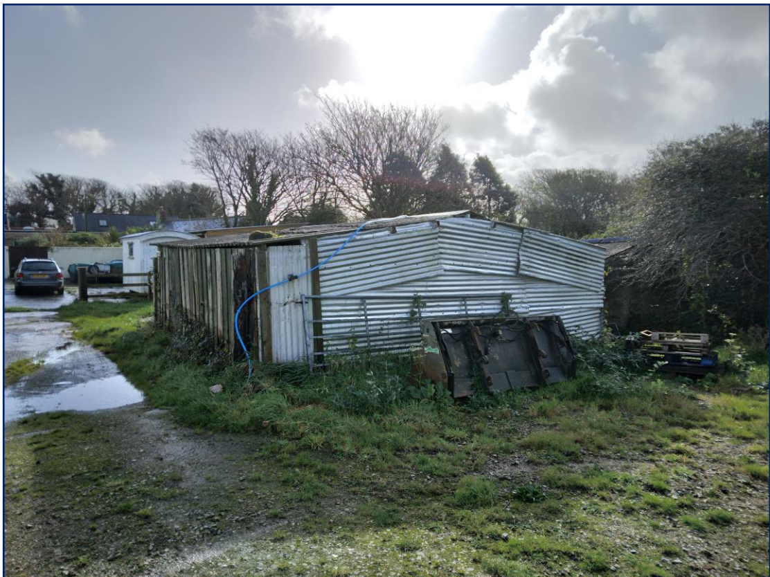
Above: existing building.
