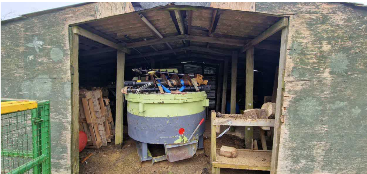
View inside building.
