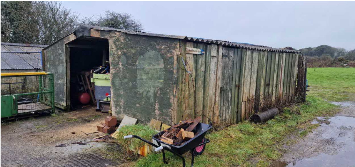
Exterior of building.
