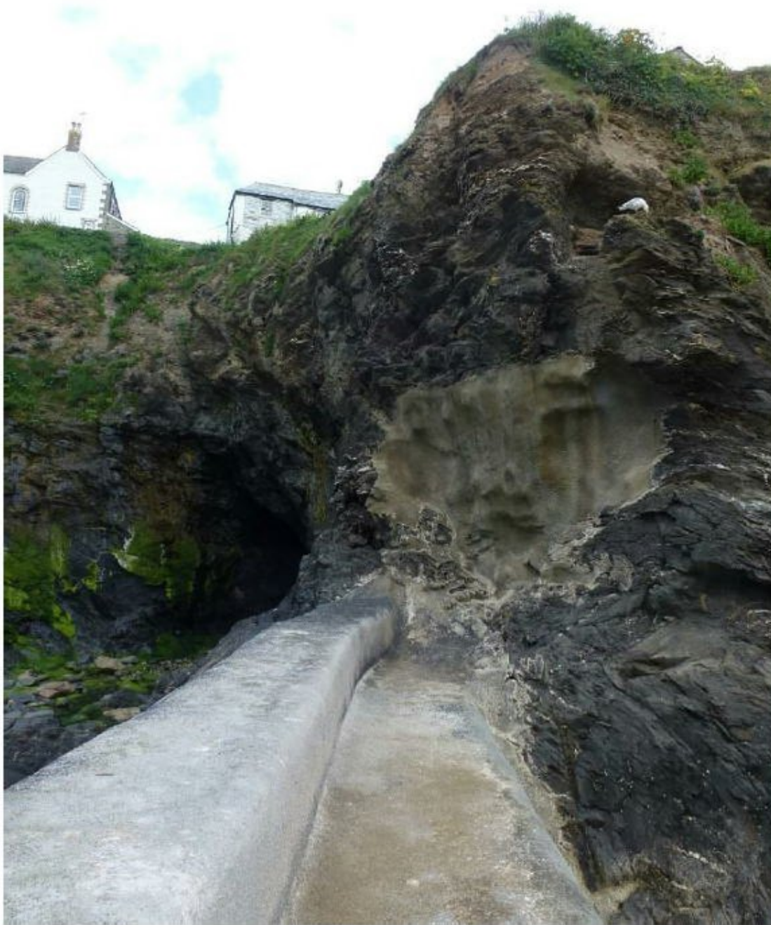
Photograph 12 – Breakwater with north face beyond
