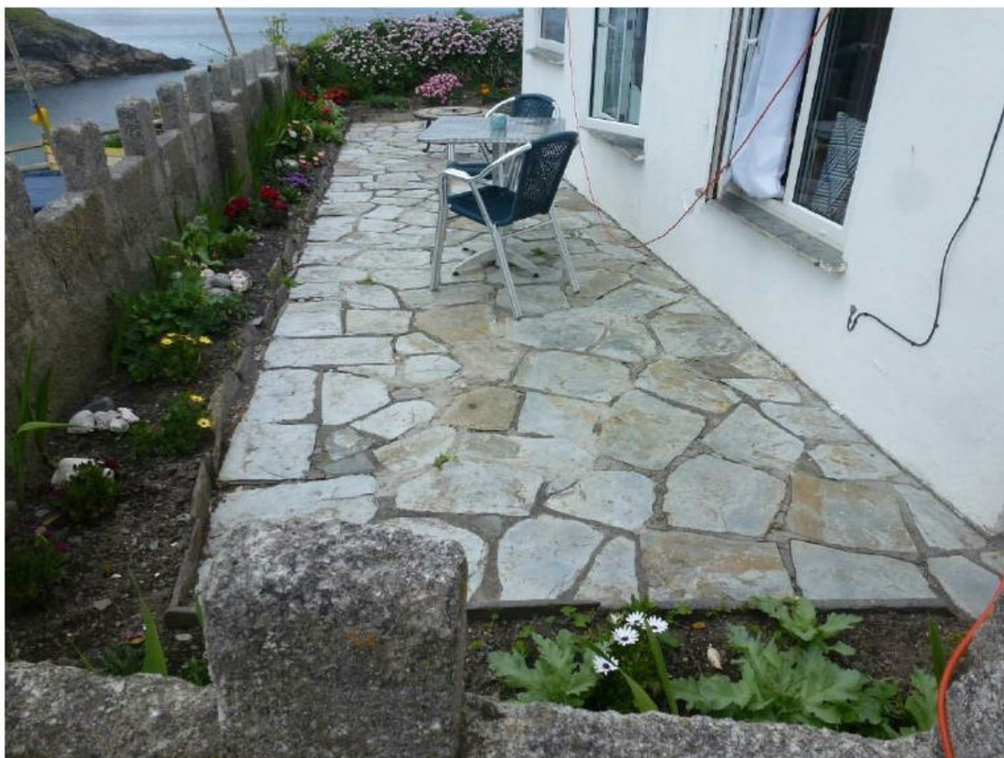
Photograph 5 – Footway in front of property in relatively good condition
