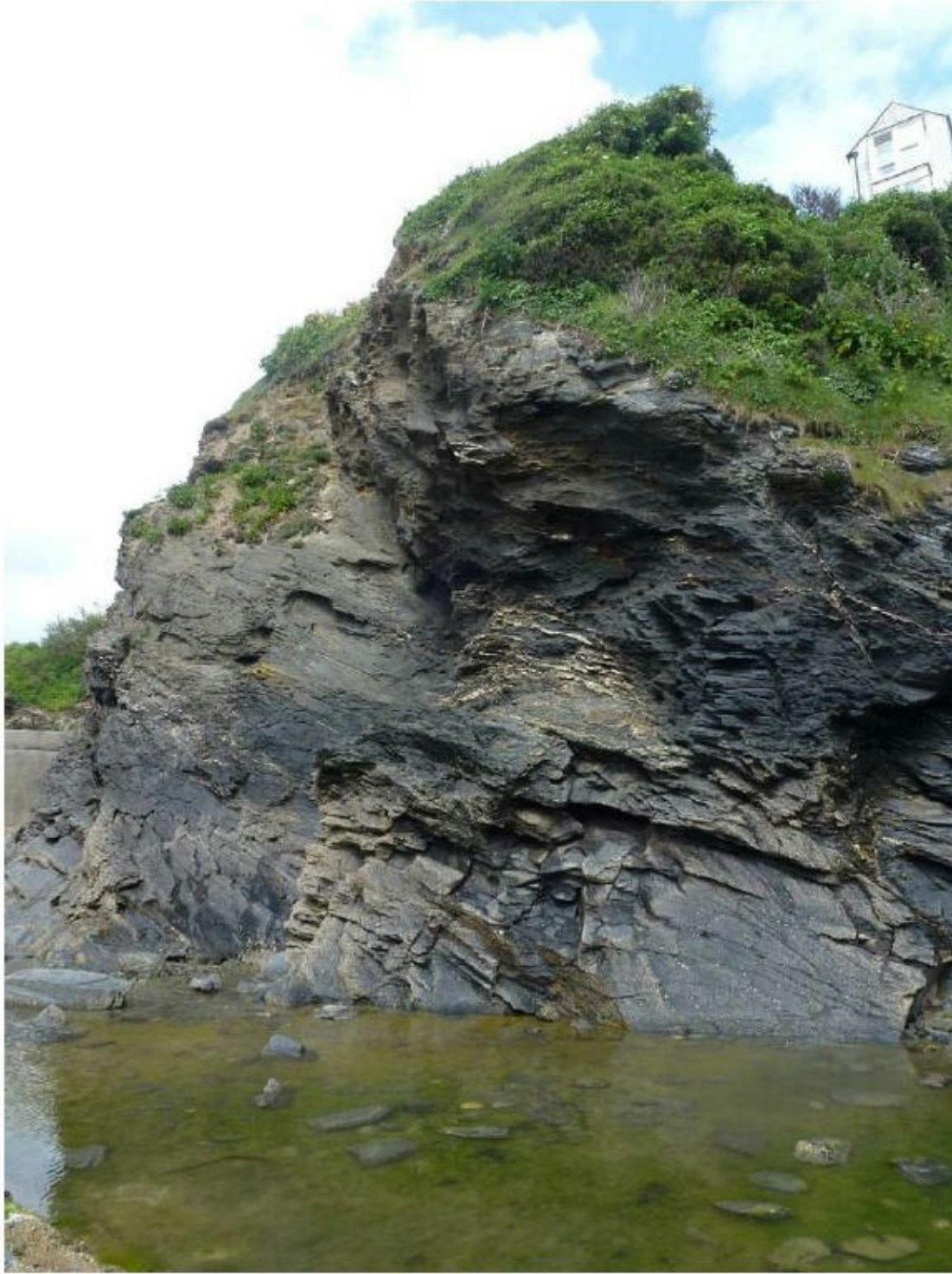
Photograph 10 – Northern eastern face
