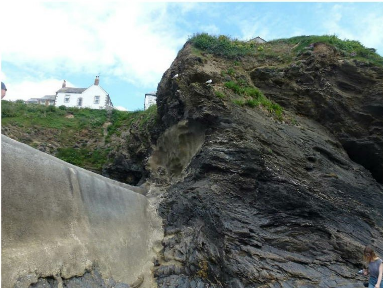
Photograph 11 – Western face showing rock outcrop and concrete breakwater to the left
