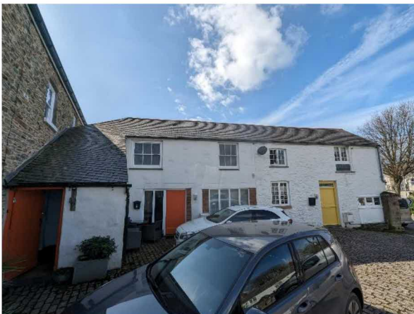
Photo 1. Showing the building from the east
