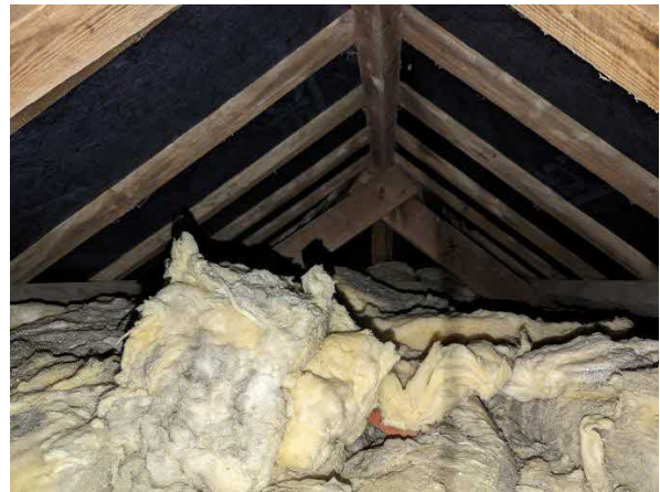
Photo 4. Showing the roof void over the northern end of the building
