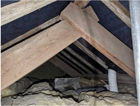
Photo 3. Showing the roof void over the southern end of the building
