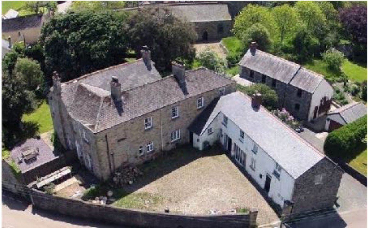
The Old Vicarage, Churchtown, St Newlyn East, Cornwall, TR8 5LJ
