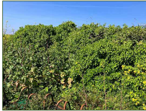
Photograph 7. Vegetated stone wall in the eastern corner
