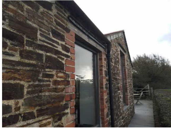
Photograph 2 – View of the south gable end.
