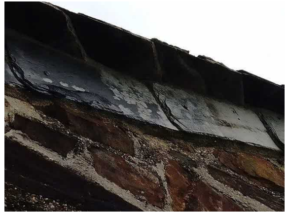
Photograph 4 – View of the sealed edge tiles on the south gable end.
