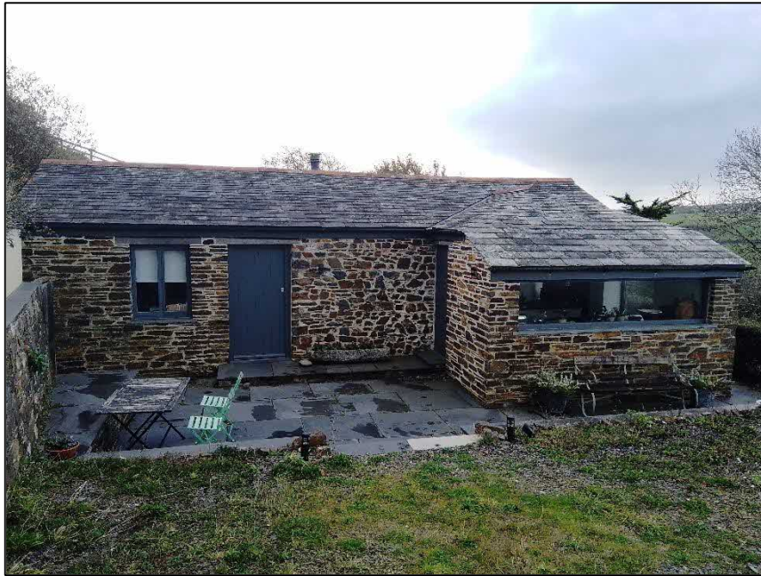
Photograph 1 – View of the west aspect.
