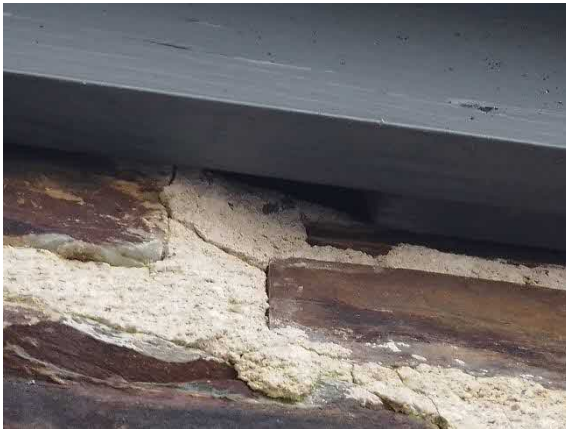
Photograph 3 – Example view of bargeboard gaps that were inspected via endoscope.
