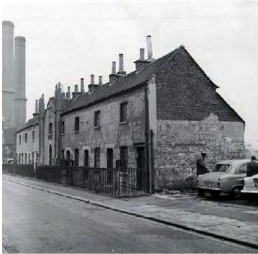
Plate 7: Ropeyard Rails photographed c.1958 just prior to demolition
