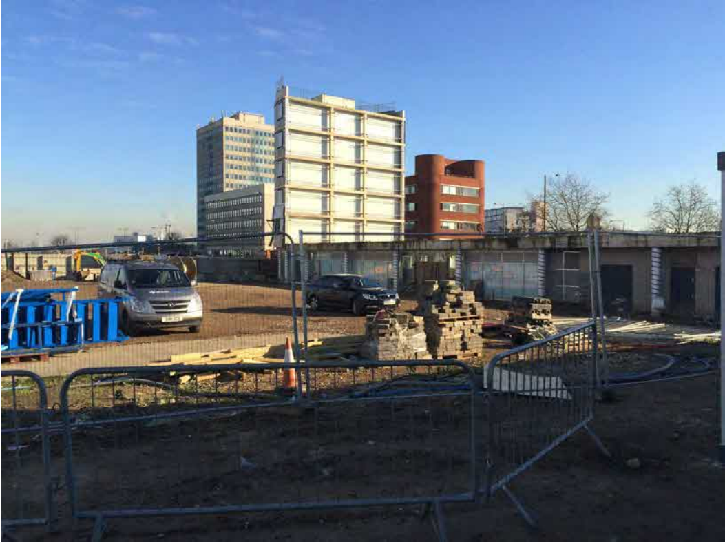
Photograph 7: View of hotel section of the site facing north.
