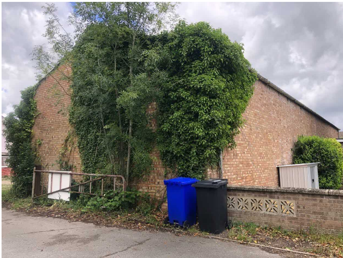
Photo 14, south and east aspect of building two, looking northwest.
