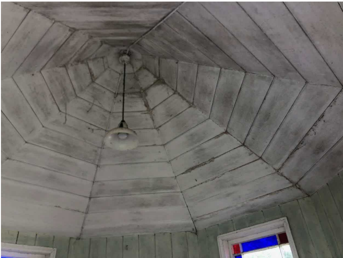
Photo 17, internal view of building three.
