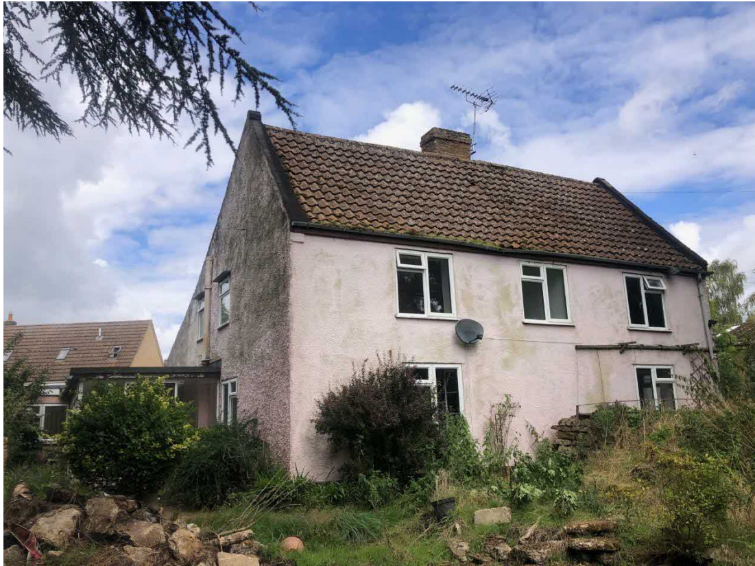
Photo 10, south and west aspect of building one, looking north.
