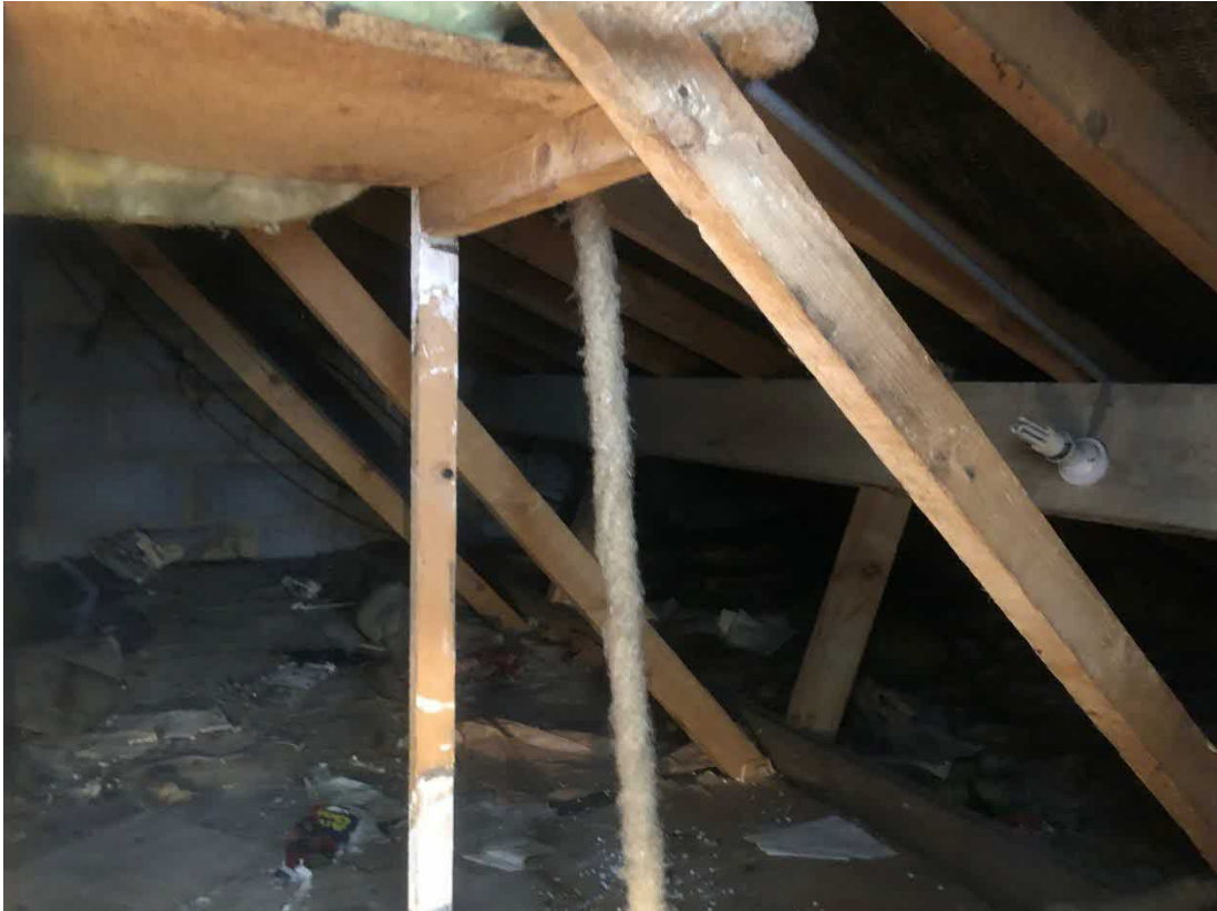
Photo 12, internal view of building one (dwelling 2a) loft space, looking west.
