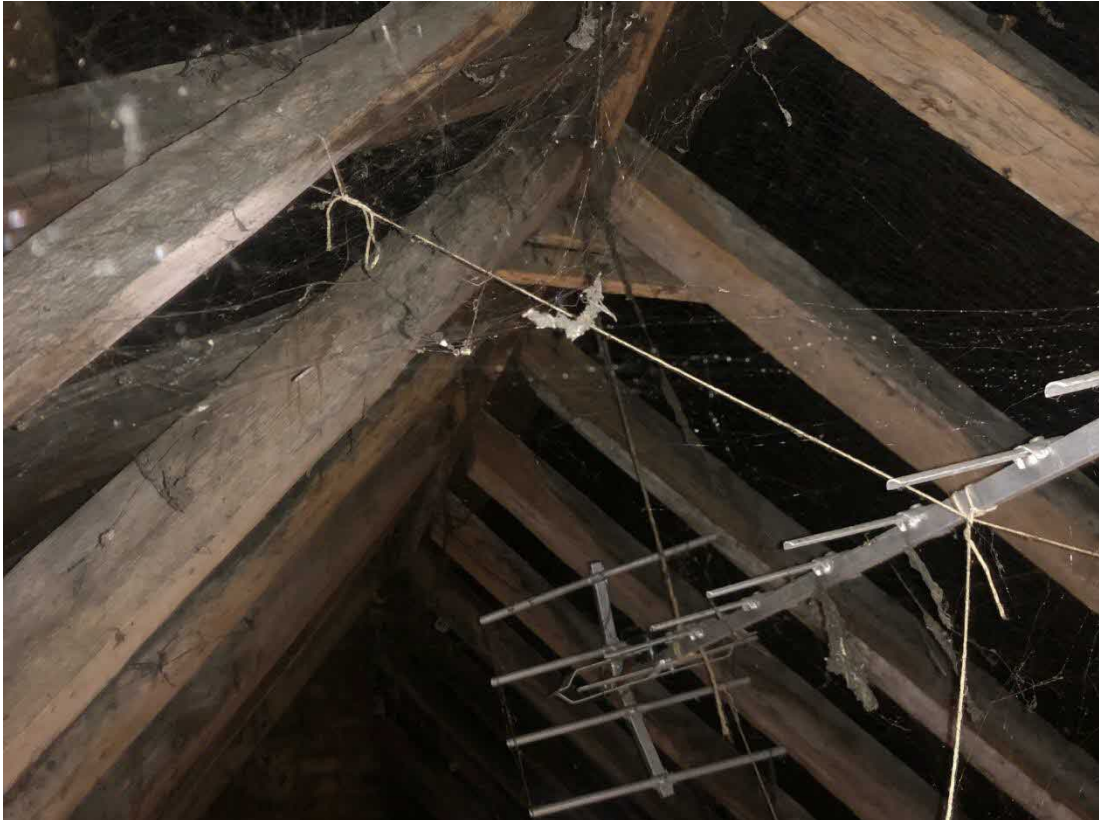
Photo 13, internal view of building one (dwelling 2b), looking west.
