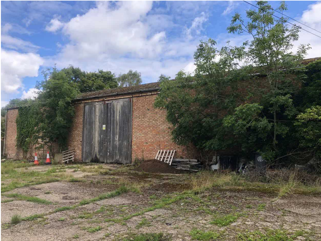
Photo 14, western aspect of building two, looking northeast.
