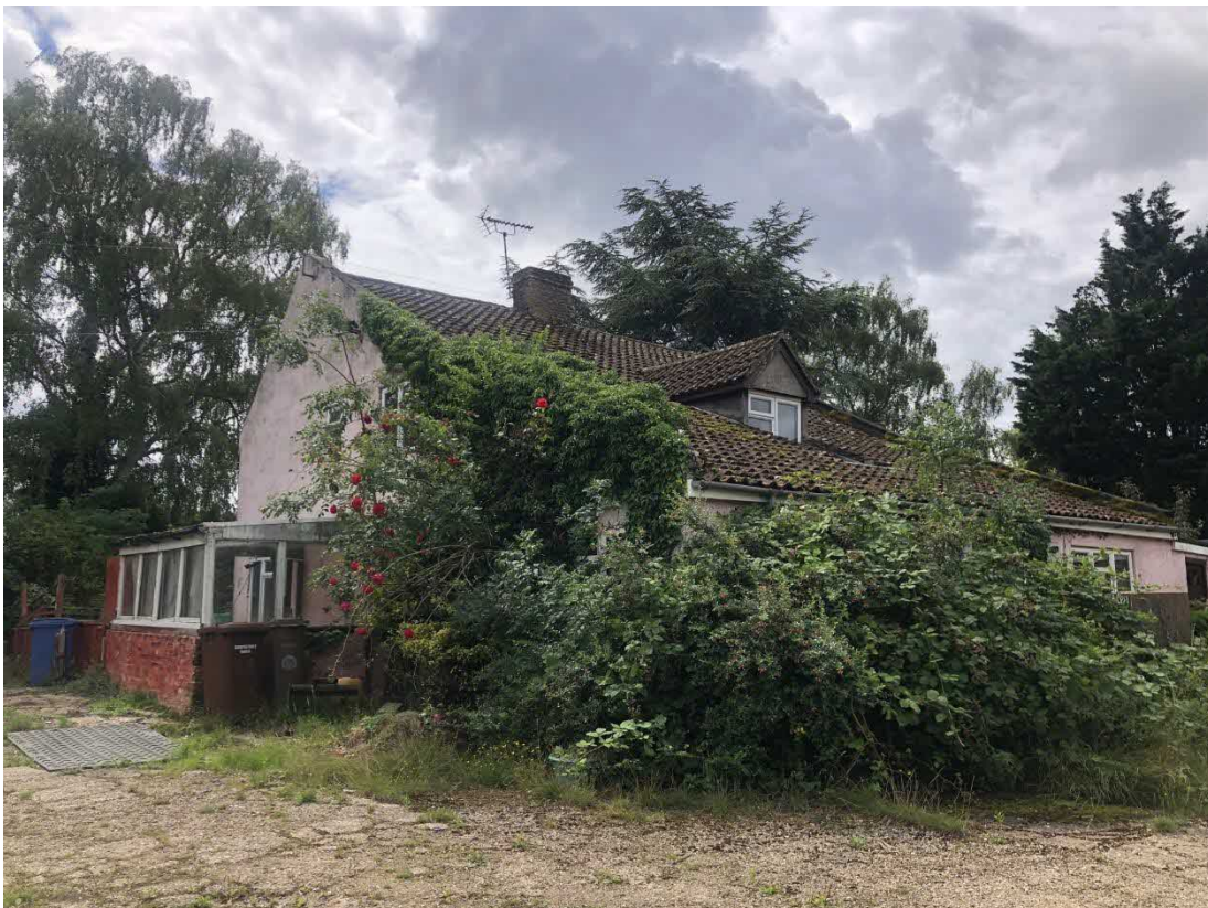
Photo 9, north and east aspects of building one, looking southwest.
