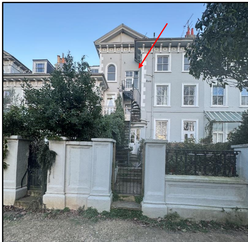
(The rear elevation of the fire escape)
