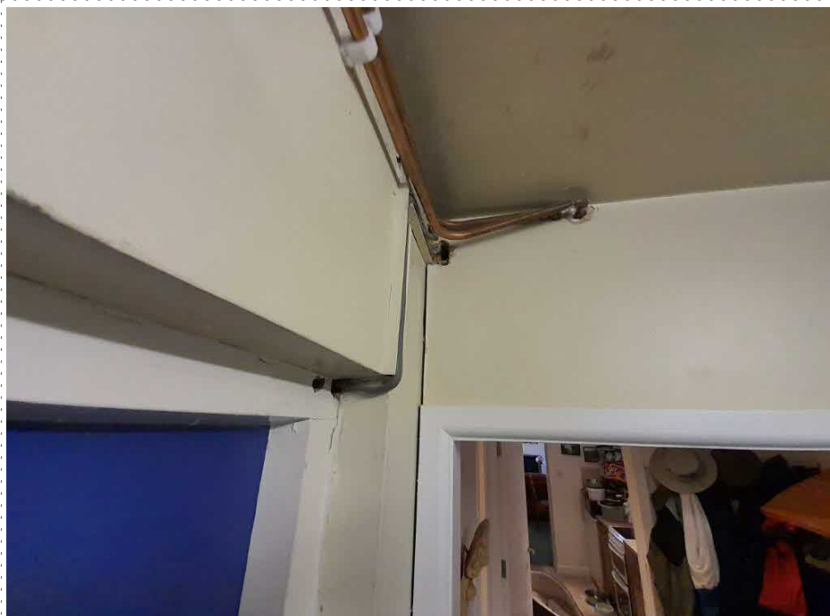
Plate 14. Vertical crack to rear wall of garage/workshop at junction with original property.
