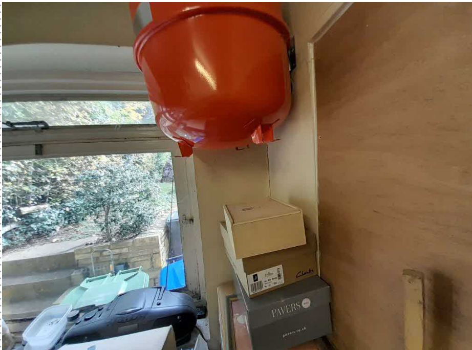
Plate 13. Vertical crack to front wall of garage/workshop at junction with original property.
