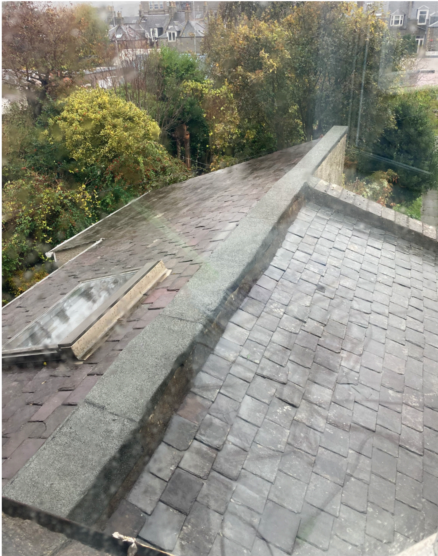
Rear of existing extension to West. Looking to roof of number 48.
