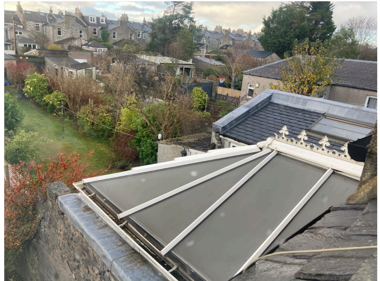
Rear of existing extension to West. Looking to roof of number 44
