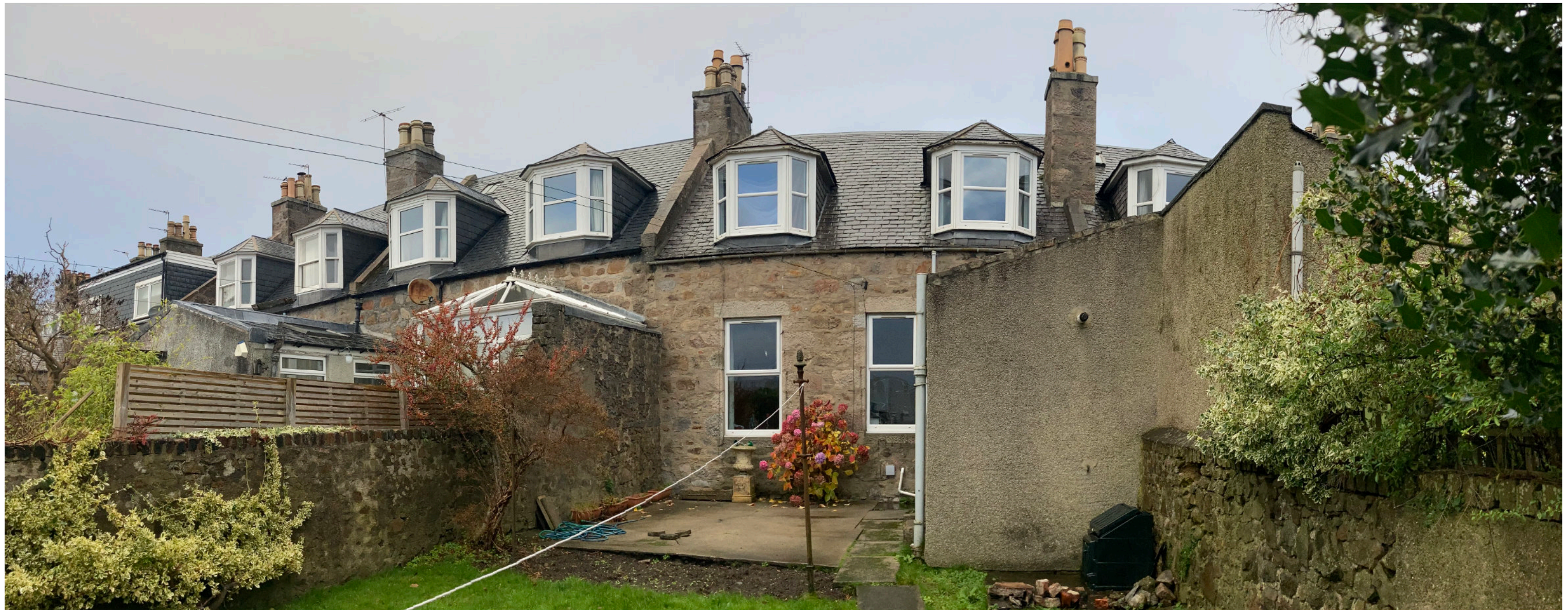
South 'Principal' Elevation - Note existing extension to West.
