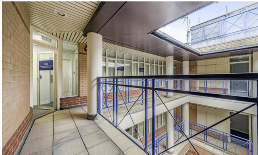
Below: Second floor access balcony, looking towards unit.
