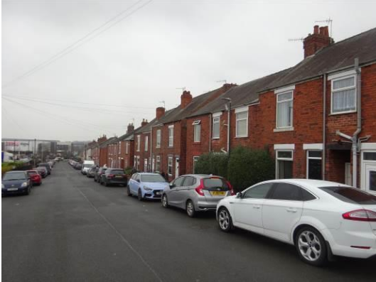
Residential terrace to Lockoford Lane
