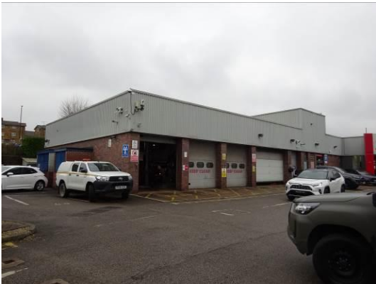
Existing gable frame to be demolished south east elevation
