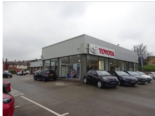
Existing south east / north west elevation To showroom
