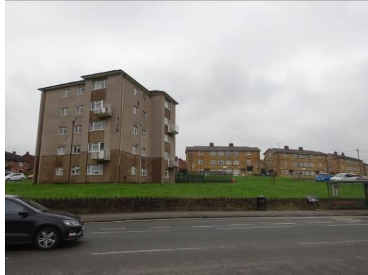
Residential flats to north west
