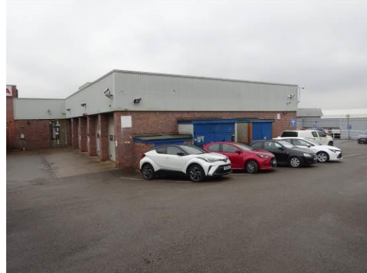
Existing gable frame to be demolished north west elevation
