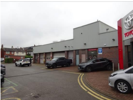
Existing south east elevation to workshop
