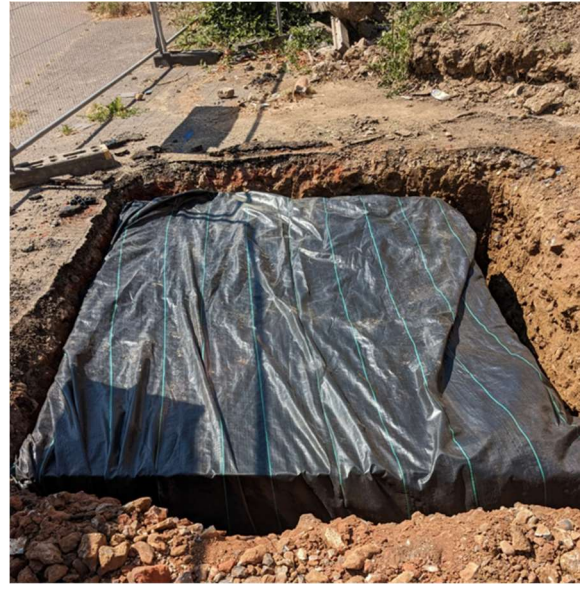
Soakaway SA2 Installed
