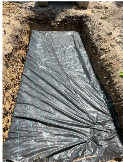
Soakaway SA1 Installed
