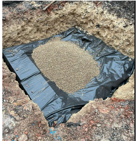
Soakaway SA4 Installed
