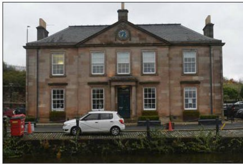
Plate 6: Canal House, Speirs Wharf (CHS 5).
