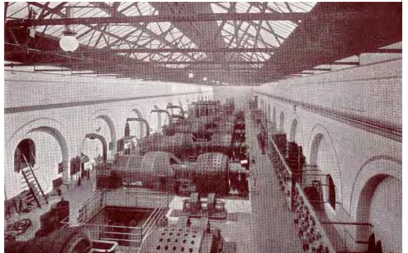
▼ Port Dundas Power Station at New Rotterdam Wharf
