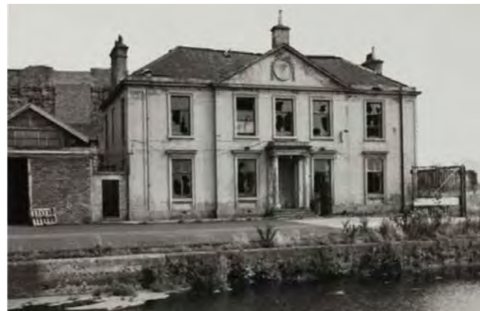
From top: RCAHMS images View of Speirs Wharf warehouses looking north from west bank of canal. Ref SC 2140013 View of southern end of Speirs Wharf warehouses Ref SC 2543652 View of Canal House, offices for Forth and Clyde Navigation Company Ref SC 2543678
